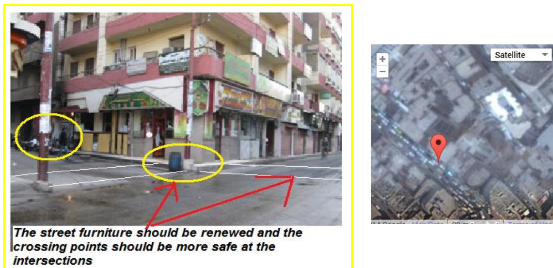
Figure 6.94: Removing the deteriorated streets furniture and providing the intersections with traffic light and safe crossing areas is proposed to improve Thabet Street
