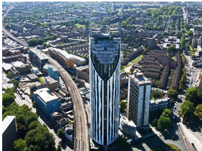
Figure 3.9: The perception of built objects through the over-head images. “The Razor”, the 148 meter-tall Strata tower topped with a trio of turbines that produce power, London, UK ( http://inhabitat.com/tag/london )
