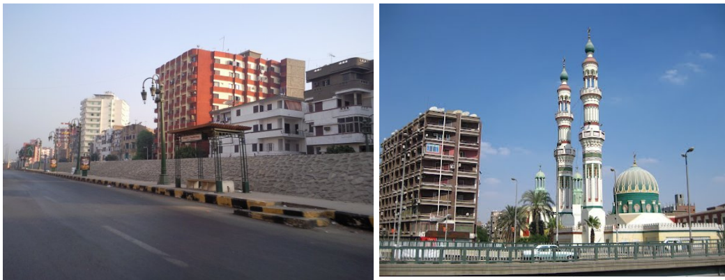
Figure 6.48: Left: Modern towers and street furniture are the main features of Al-Geish street ( http://www.panoramio.com ). Right: Al-Geish Bridge occupies Al-Geish Street to reduce the traffic cognition in this street which is one of the approach axes to Assiut University.
