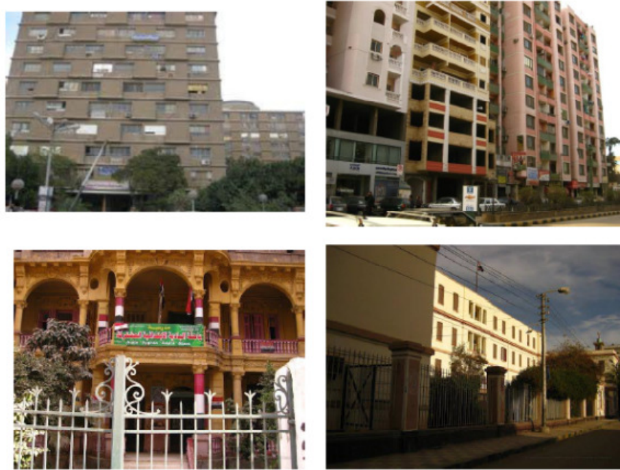
Figure 6.32: Above left: The Complex of Governmental Services, right: The commercial and residential uses. Bottom left: Bahethat Al Badia School, right: Khadega Yousef School ( www.panoramio.com )
