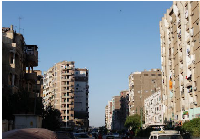
Figure 6.65: The visual effect of tall buildings in closing the view from the street and reducing the legibility of the surrounding historical buildings.
