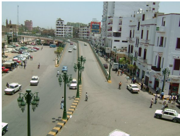
Figure 6.42: The entrance of Al-Helaly Bridge from Al-Mahata Square going to the East
