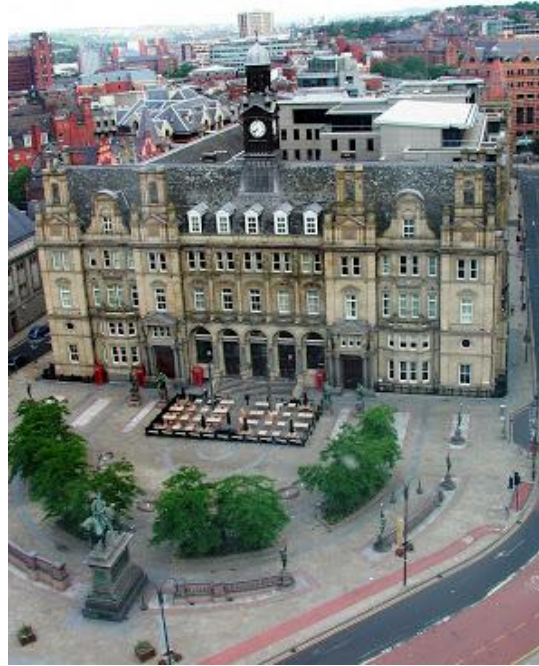
Figure 4.15: The Old Post Office Building, Leeds City Centre. The open space, street furniture and the statue in the front of the building have a great effect on highlighting this old building to be not lost in the image of the city centre ( www.aireboroughcivicsociety.org.uk ).
