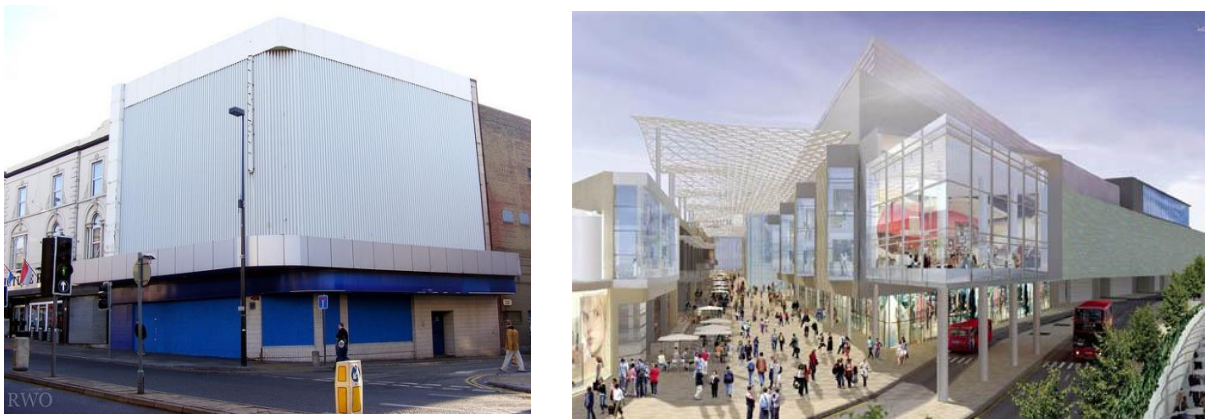
Figure 3.10: A comparison between the visual effect of the passive facades and the active frontages on the image of buildings from the street level. Left: Leisure parade in Liverpool, UK ( http://farm4.staticflickr.com ) and right: Shopping centre in London, UK ( http://www.whats-on-in-london.com )
