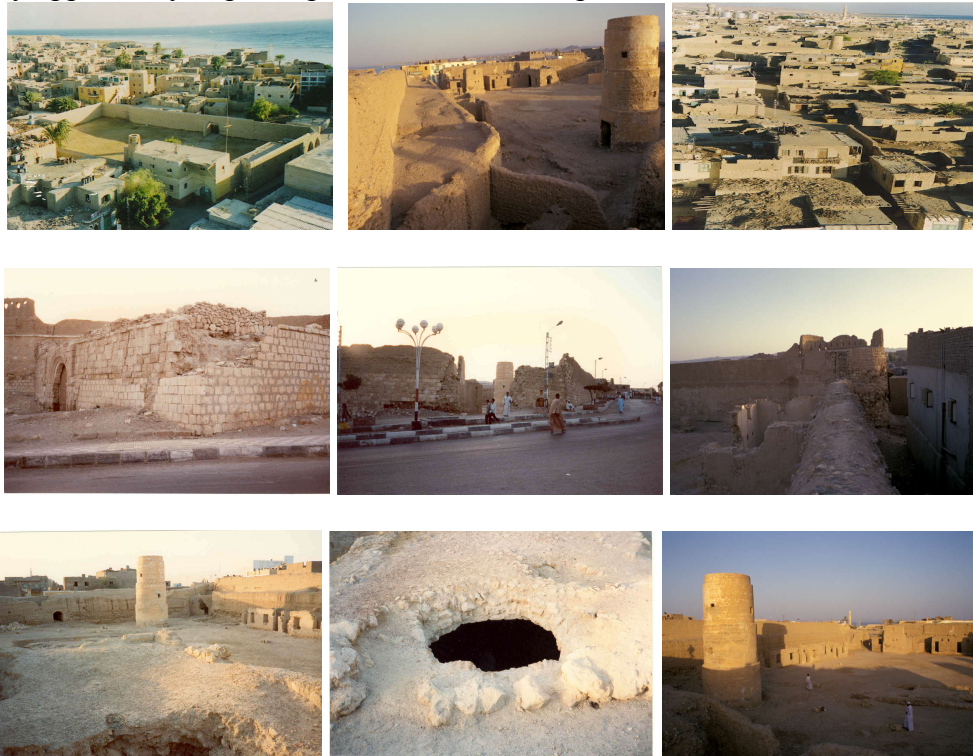
(Figure 1) Photos showing the fort before the restoration project
