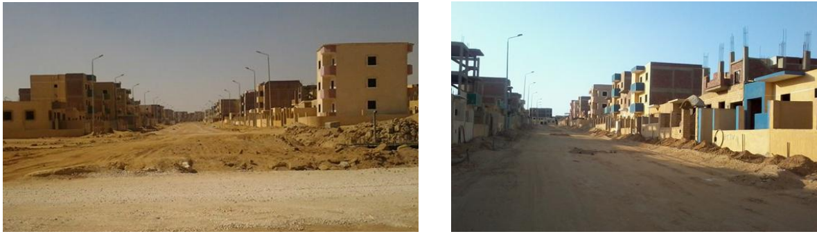
Figure 2. “Build your Home, Ibni Baetak ”, 6 October New City, Egypt – advanced implementation of the “Private Product”: Dwellings on Plots.
