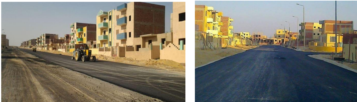
Figure 3. “Build your Home, Ibni Baetak ”, 6 October New City, Egypt – current status, advanced implementation of the “Private Product”: Dwellings on Plots and late completion of the “Public Product”.
