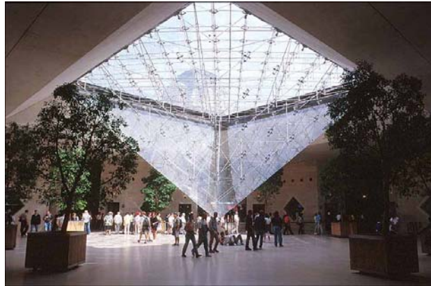
Fig (3-65): the “ Pyramide Inverse ” at the “ Carrousel du Louvre ” used to provide daylighting to the underground commercial center entrance.
