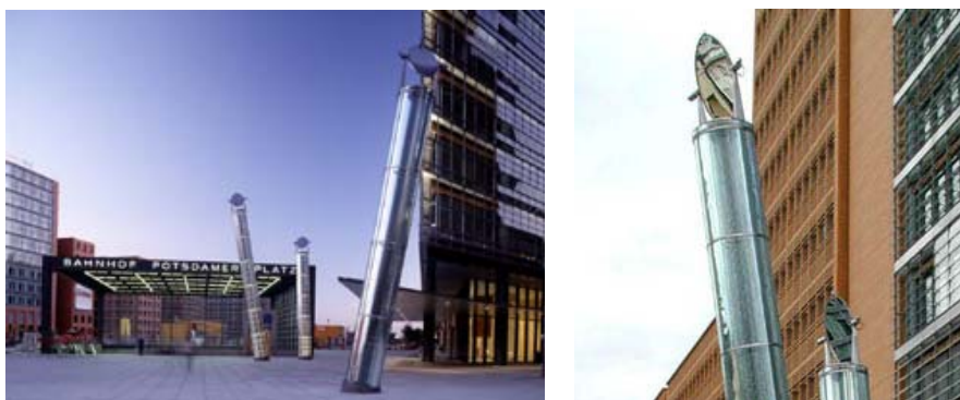
Fig (4-54): Light pipes on Potsdamer Platz in Berlin, Germany.
