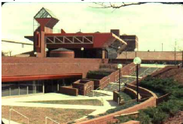
Fig (4-9): The Civil and Mineral Engineering Building (an example of the mid-scale system is the passive system used in this building).
