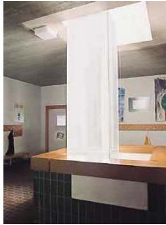
Fig (4-28): The light guide tube illuminating the core of the building
