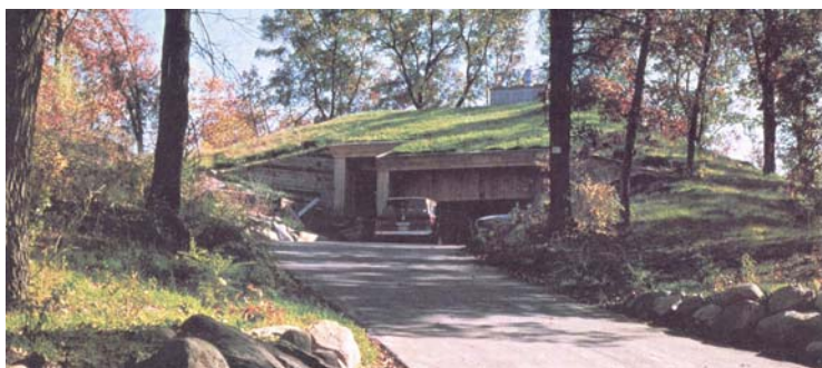
Fig (1-15): Burnsville house, Burnsville, Minnesota (1) .
