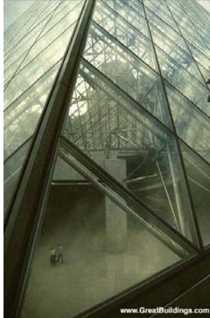
Fig (3-62): The glass pyramid glazing detail showing the aluminum frame and the clear glass used.
