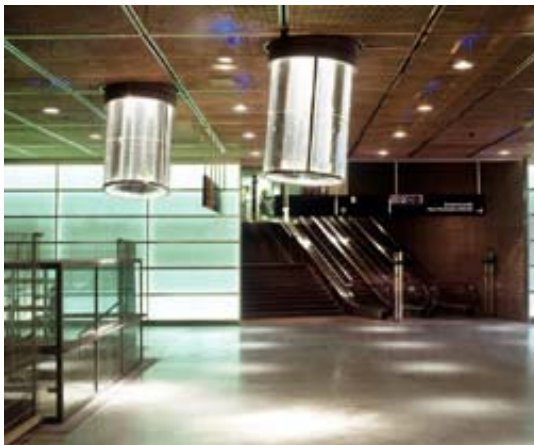
Fig (4-56): Interior view of the light pipes end.
