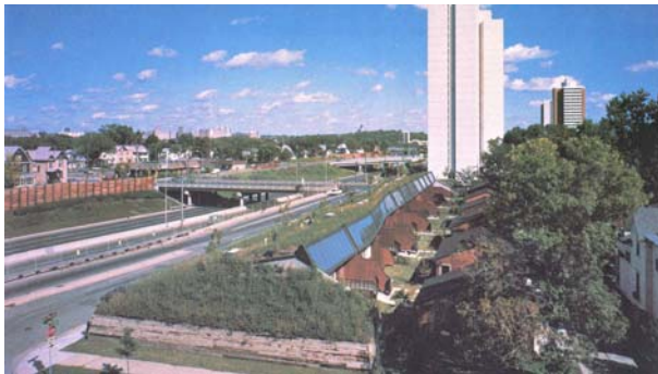
Fig (1-14): Seward town houses, Minneapolis, Minnesota.
