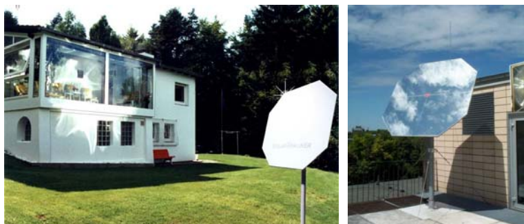
Fig (4-8): Small-scale heliostat system (garden and roof type).
