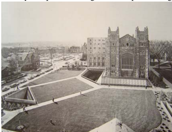
Fig (3-41): Law library exterior view from the east showing the original building and the L-shaped skylight of the new extension.
