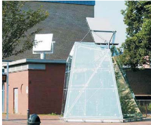
Fig (4-12): Exterior view of the lightron system showing the primary and secondary mirror.
