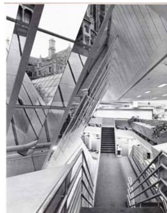
Fig (3-47): Interior view of the skylight showing the 0.9 meter mirrors on the sloped glazing
