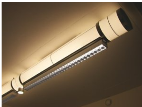
Fig (4-21): The sun-luminaire showing the longitudinal and central elements in addition to the artificial lighting.
