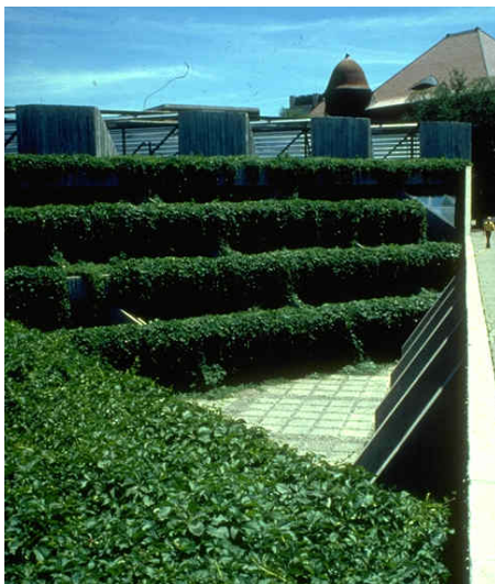
Fig (2-62): View of the court showing the tiers of planters with the Engleman ivy plants used to shade the glazing in summer.
