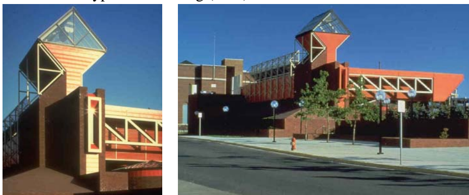
Fig (4-39): Exterior view of the cupola housing the active heliostat.
