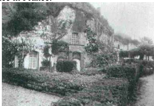
Fig (1-12): Façade of a house dug into the hillside in the Loire Valley, France (3) .
