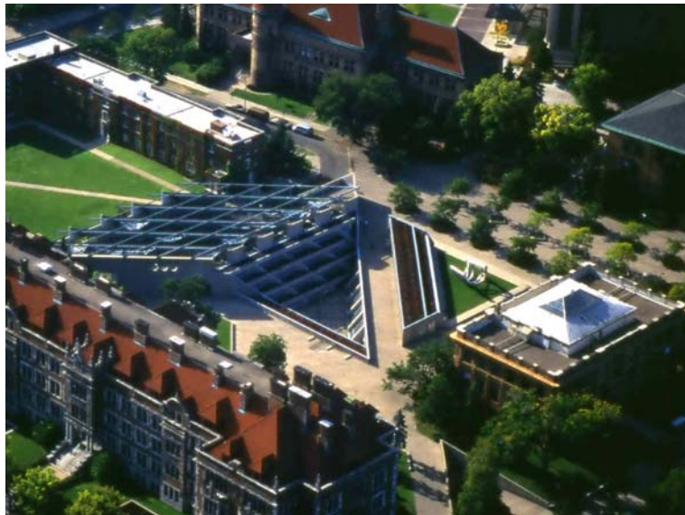
Fig (2-54): Williamson Hall aerial view showing the underground building and the historic site.
