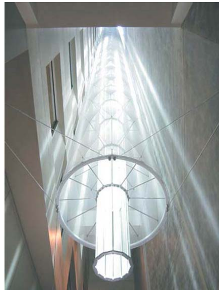
Fig (4-52): The solar light pipe.
