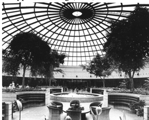
Fig (3-54): Interior view of the garden court showing the main daylighting theme - the glass dome.
