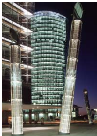
Fig (4-55): Exterior view of the light pipe at night.
