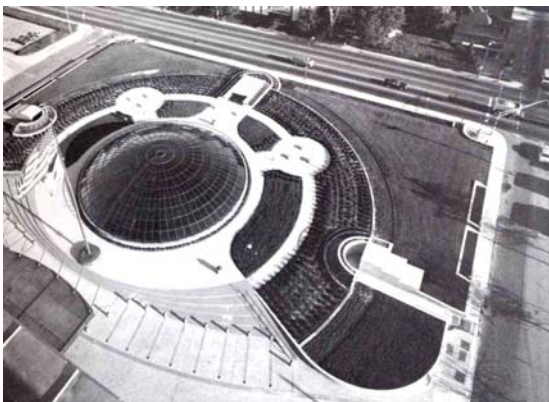
Fig (3-51): The underground addition viewed from the roof of the original headquarters building showing the glass dome.
