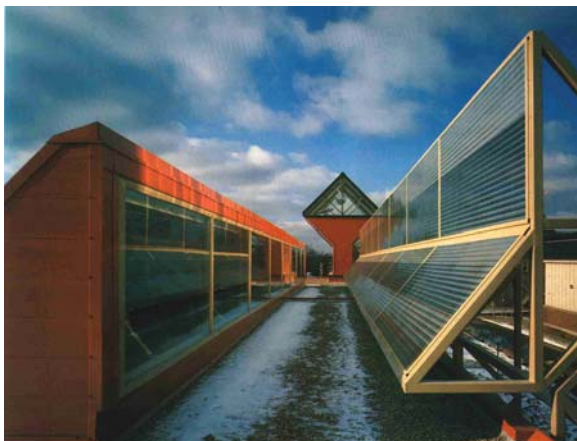
Fig (4-35): The Active and Passive heliostat systems at the CME Building.
