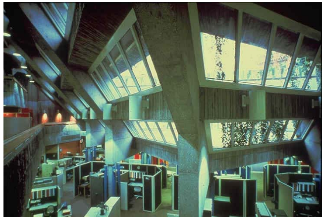
Fig (2-60): Interior view of the offices area showing the daylighting fenestrations used.
