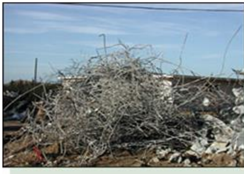
(Fig. 3) Material segregation.
