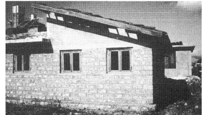
(Fig. 1) Filling the mold with rubble stones and compacting. (Fig.2) Stone masonry construction using pre cast rubble. (Stulz & Mukerji 1993)
