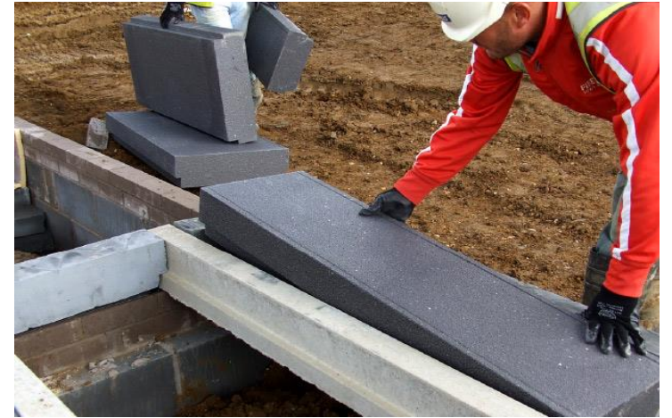
Laying Eps infill, Jetfloor blocks
