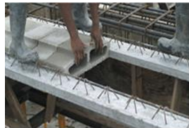
Placing blocks of "Urban Kwik" floor in Ghana
