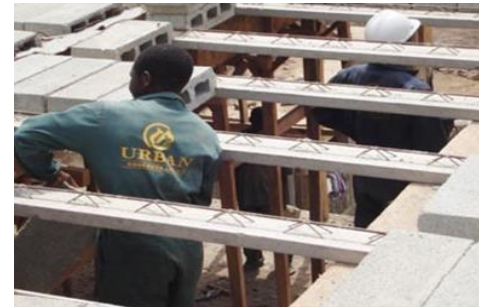
Construction of "Urban Kwik" floor in Ghana
