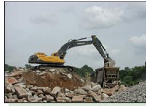
(Fig. 4) Rubble crushing.
