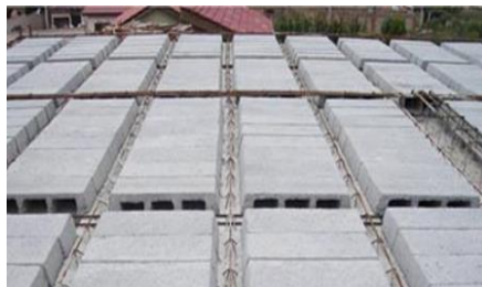
Placing blocks of "Urban Kwik" floor in Ghana
