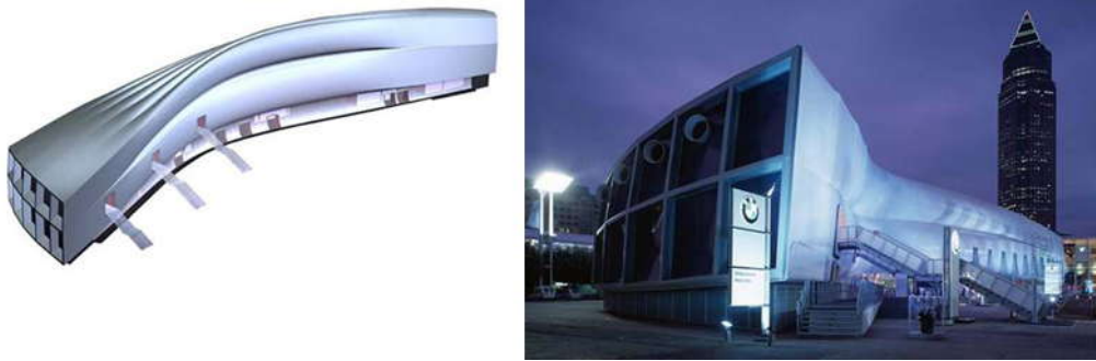
Fig. 5.41, 5.42 The "Dynaform", BMW pavilion, Auto show in Frankfurt, Germany, 2001. architects Bernhard Franken and ABB Architekten (will be mentioned in detail later on in this chapter).
