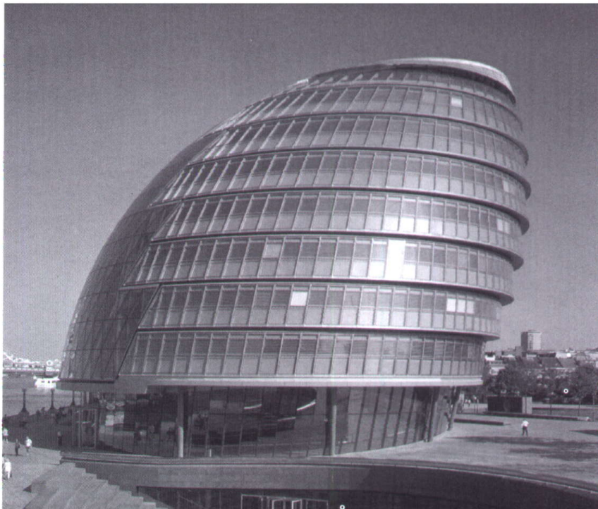
Fig. 5.129 Post nature of City Hall shows, how the glazing system was fabricated like cylinders.
