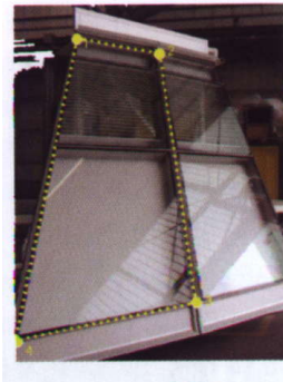
Fig. 5.130 Flat-patterned drawing of the glazing solution for city hall.
