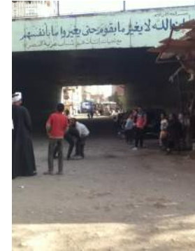
A tunnel providing access to the area
