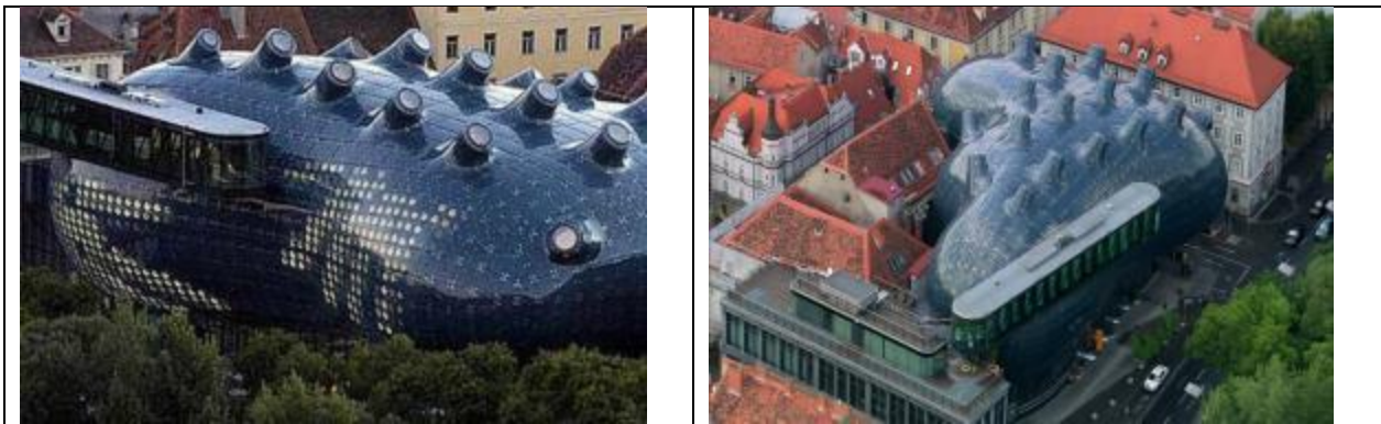
Fig.15 Kunsthaus Graz museum- Graz, Austria - designed by Peter Cook and Colin Fournier- The building's innovative complex double-curved geometric façade- an enormous biomorphic shell defined as "friends alien".
