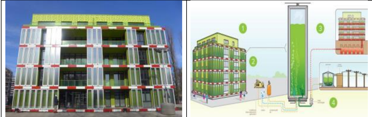
Fig.19 BIQ House -Hamburg,Germany- designed by joint venture between Splitterwerk Architects, ARUP, Colt International and Strategic Science Consult -the world's first algae powered building
