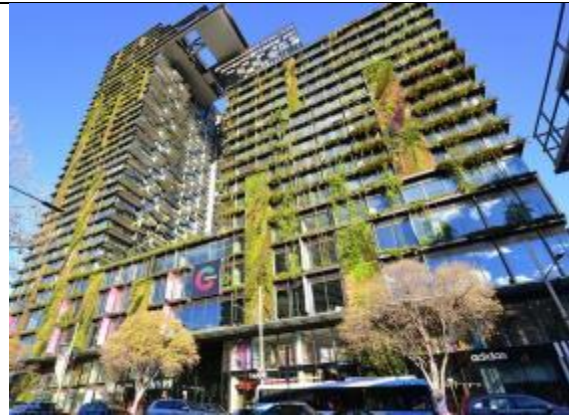
Fig.17 Central park building-Broadway,Sydney- with green walls on the exterior of a high-rise
