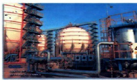
Tanks of Liquid petroleum gaz. (Spherical tanks)
