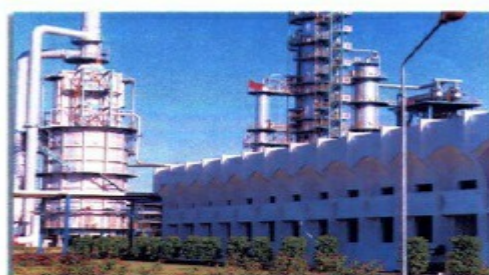
Distillation Columns Building (DCS) (Fr actionator)
