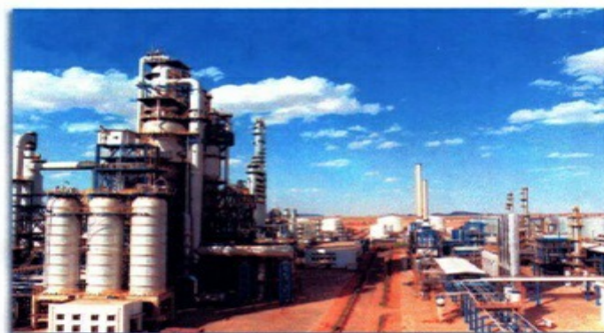
Residual oil catalytic cracking Unit (RFCC) . and Reforming Unit(REF)
