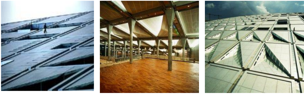
Figure (10): The tetrahedrons in the ceiling act as passive solar convectors, pulling cool air if the electrical and mechanical systems failed.
