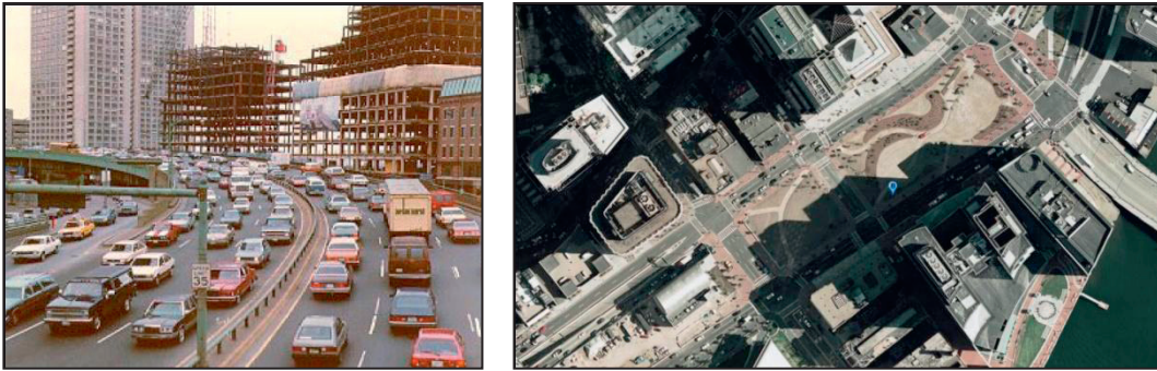
Fig. 3. Boston John Fitzgerald Expressway - Central Artery, before & after the project (Source: BECT/AREP, 2009)
