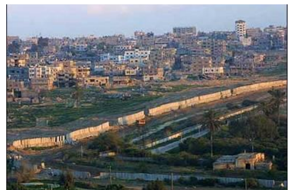
Fig 10: The high population and building densities of the Palestinian Rafah contrasted with the Egyptian one.
