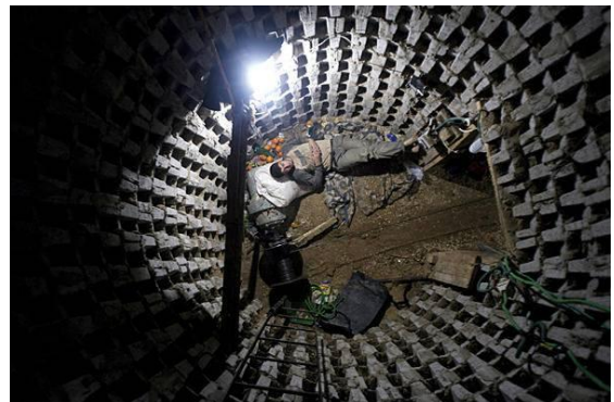
Fig12: The tunnels across Rafah are in many cases well-constructed and reinforced.
