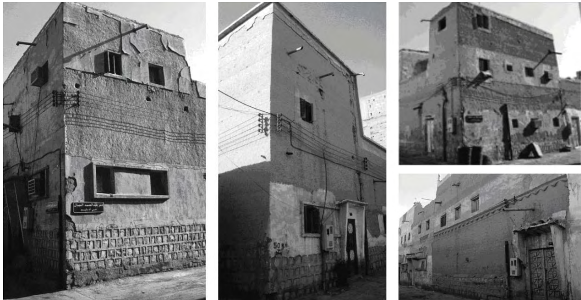
Figure 9: The mud surfaces in the traditional houses in Riyadh plastered by cement and the traditional house gate was replaced by a concrete one because it reflects modernity. (Source: Author 1995).
