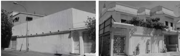
Figure16: Two villas in Hofuf (people altered the facades of their houses to provide more privacy for the front setbacks by using metal sheets to increase the height of their house fences). (Source: Author, 1995).
