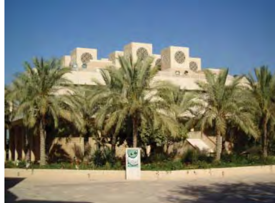
Figure 4.a: Utilization of Wind Towers in Main Administration Building of Qatar University. (Source: Author).
