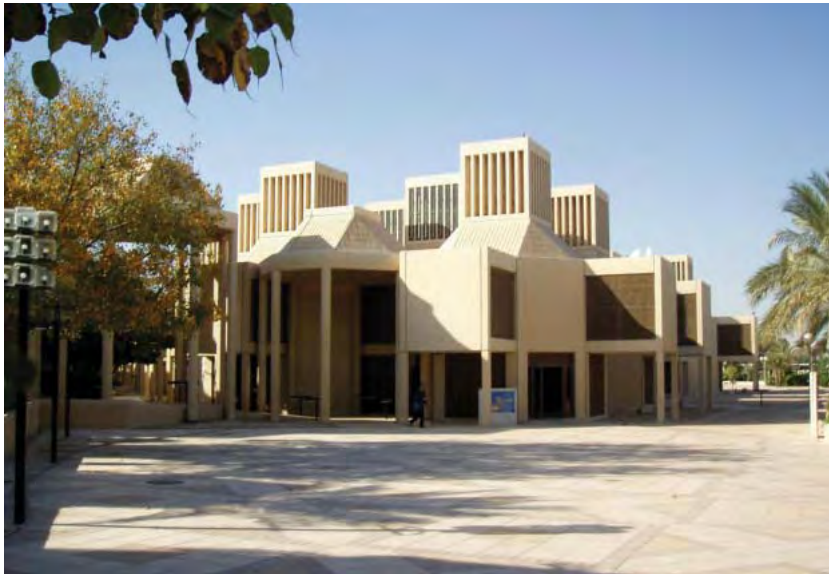
Figure 2: The Use of Repetitive Pre-cast Elements for Both Cladding and Structural Walls, A Major Design Feature that Characterizes the Design of All Educational Buildings. (Source: Author).
