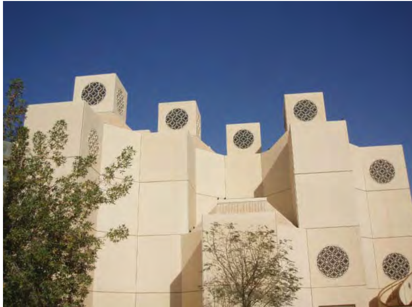
Figure 4.b: Emphasizing Natural Ventilation by Using Wind-Towers in the Education Technology Center. (Source: Author).
