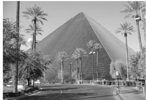
Figure 6: Luxur Hotel in Las Vegas, Nevada, the Largest Glass-Enclosed Open Atrium in the World (Source: Author).
