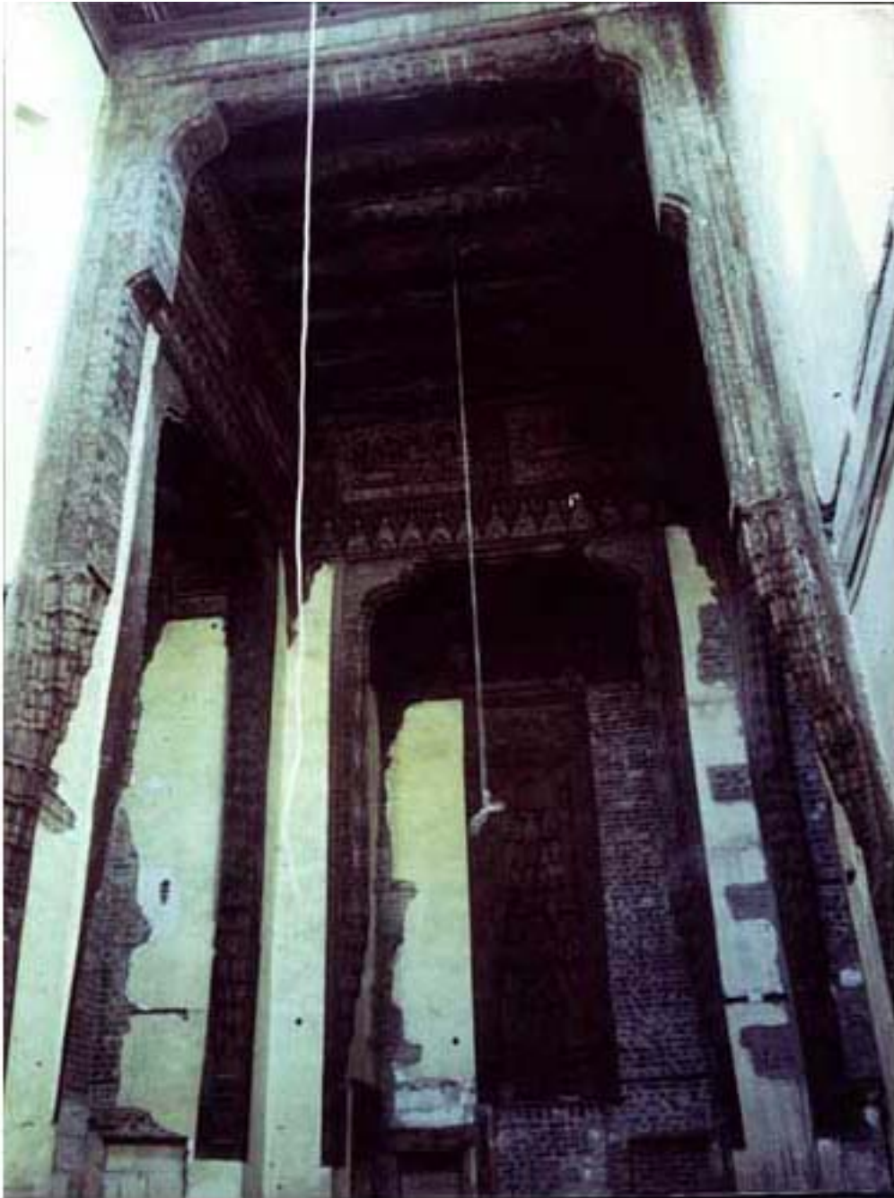
Figure 3: The Mamluk part (the original) of the Qa'a of Zaynab Khatun, Al-Azhar, Late 15th century. The exhibited lofty proportions and decorations, especially the wooden brackets and ornamented friezes and ceiling, are very characteristic of the Mamluk Period especially of Qaytbay's Reign.
