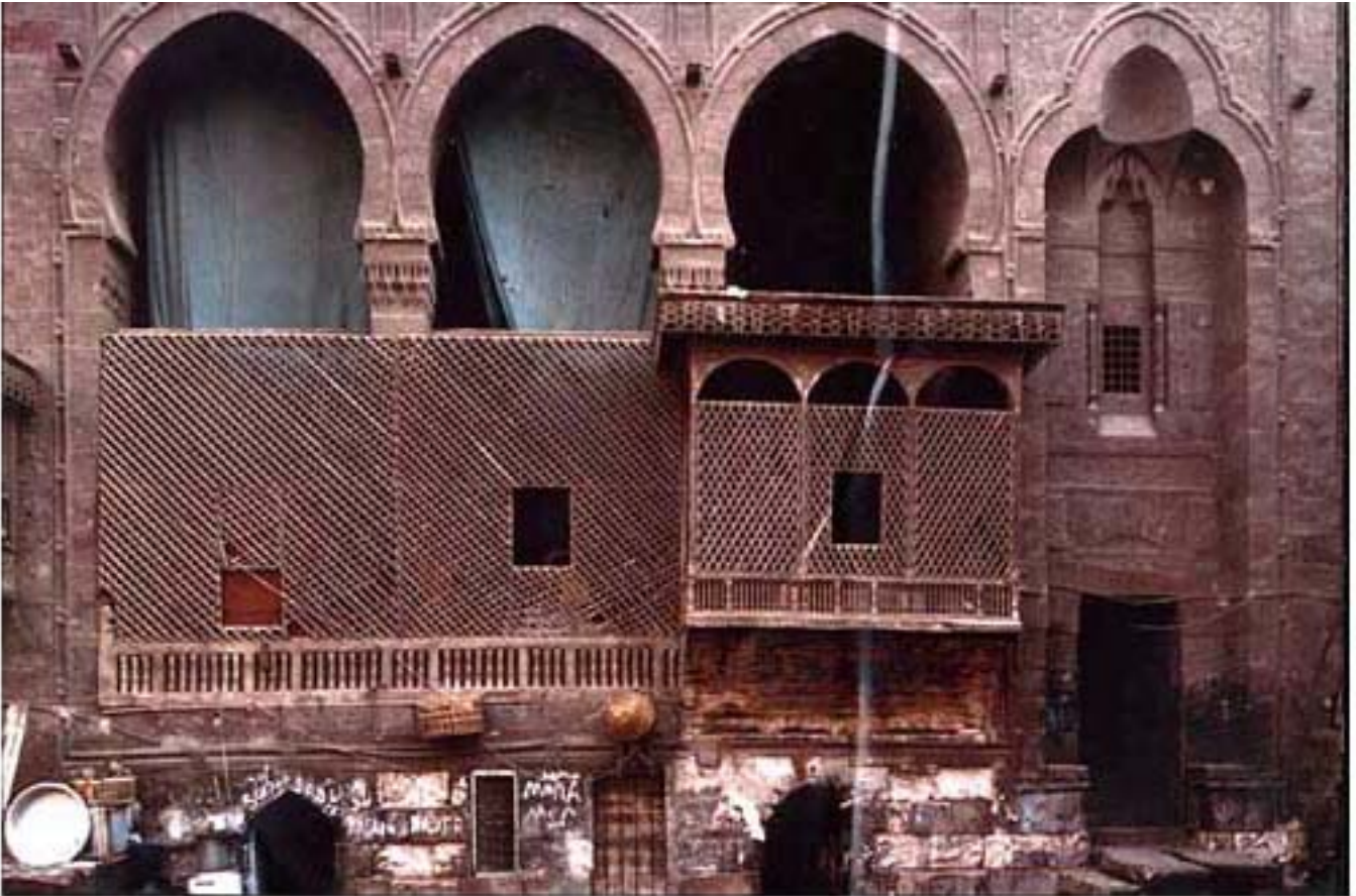
Figure 2: The 3-bay Maq'ad of Qaytbay, Maradani Street, al-Darb al-Ahmar, late 15th century. An example of the wide loggia during the Circassian Mamluk period Photo by Prof. B. O'Kane
