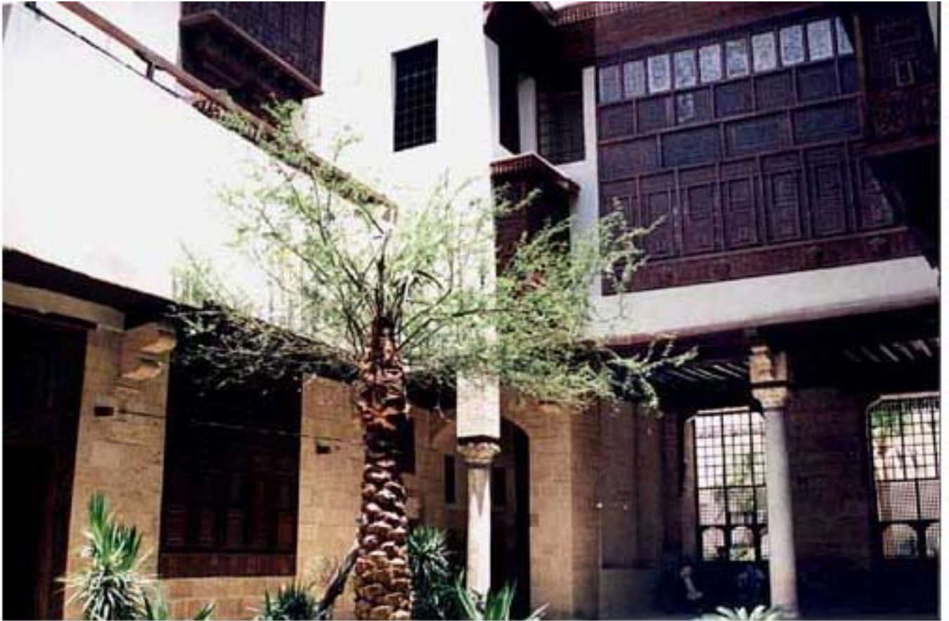
Figure 5: The Takhtabush of Al-Suhimi House, Al-Darb Al-Asfar Alley, Gamaliyya, ca. 18th century. A typical element in the court of the Ottoman house in Cairo Photo by Arch. A. Hassaballah
