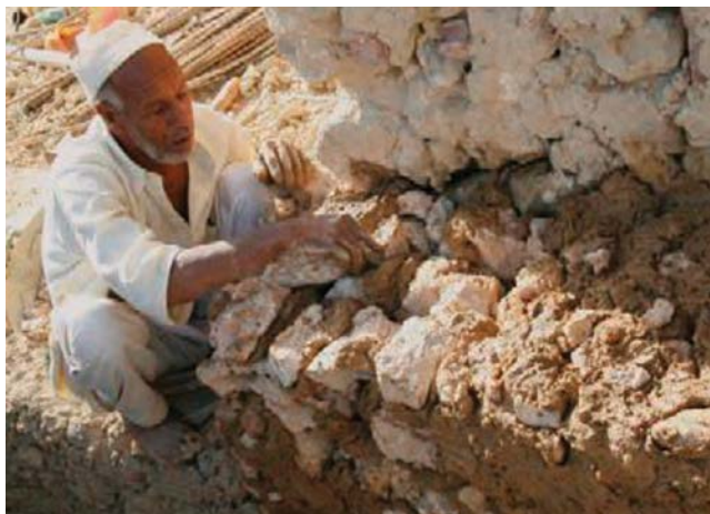
Figure 3-9. The technique of constructing the karshif wall (Calogero Montalbano, 2011)
