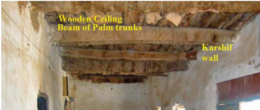
Figure 3-7. Details A, showing the wooden ceiling (The author)
