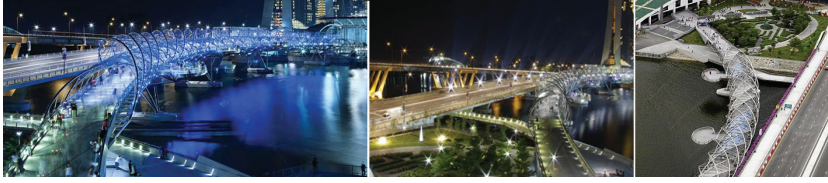
Fig. (9): Helix-bridge (www.livingpod.com/lifestyle/architecture/double-helix-curved)
