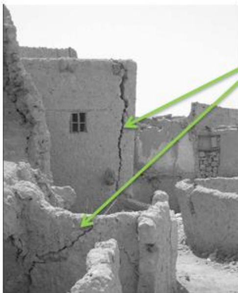
Figure 10: The cracks in the wall, Siwa, Egypt
