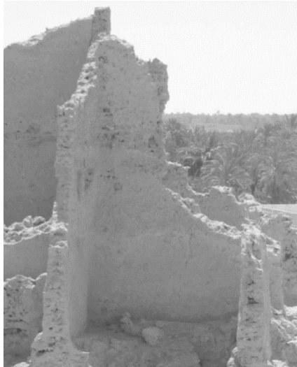
Figure 6: The wind effect on an Adobe wall, Siwa, Egypt,
