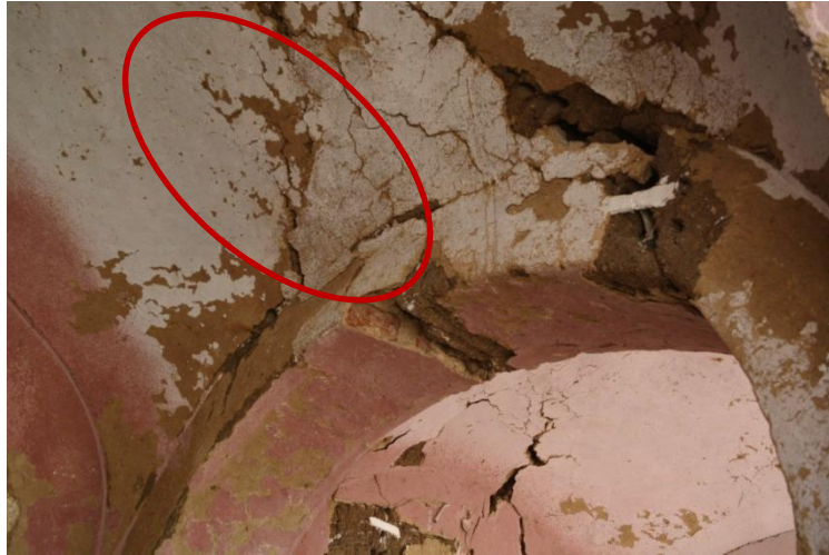
Figure 9: Adobe Disintegration, El.Qurna- Luxor, Egypt, Taken by Author
