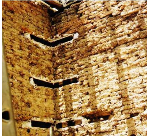
Figure 12: timber beams at the corner of adobe wall
