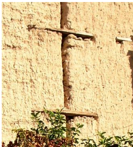
Figure 11: Installation of timber beams for the treatment of a vertical discontinuity
