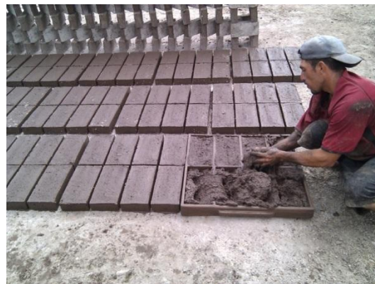
Figure 14: the framing process
