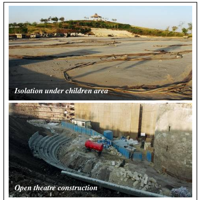
Fig. 6 Construction stage in Al-Azhar Park 35
