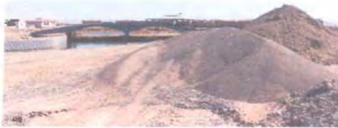
Fig. (7-67) Construction materials mixed with site excavation
