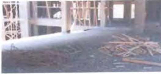
Fig. (7-53) Construction waste segregated (steel bars & wood)
