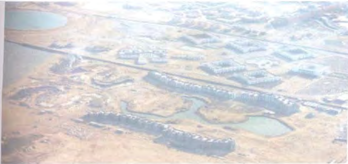
Fig. (7-64) Aerial view for the site during the construction phase
