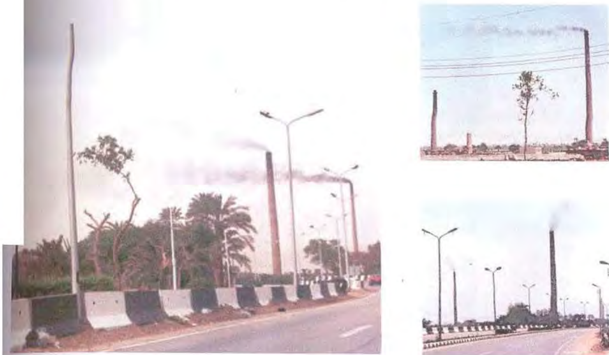
Fig (6-7,8 & 9) The effect for bricks kilns on the environment
