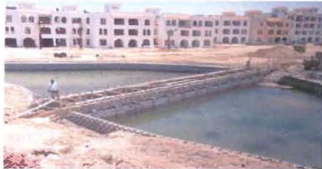
Fig. (7-68) Keystone used in construction
