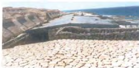
Fig. (7-36) Building roof with finished heat insulation from the dry rocky corals produced from site excavations
