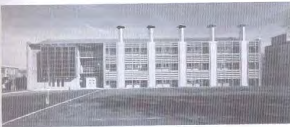
Fig 4.19 Environment Building façade with the stack-effect ventilation Source: Environmental Design- (1999)
