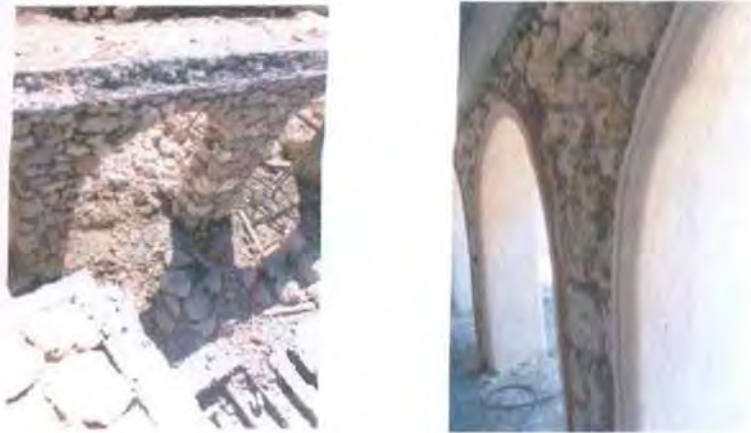
Fig. (7-34 & 35) Local materials used on site
