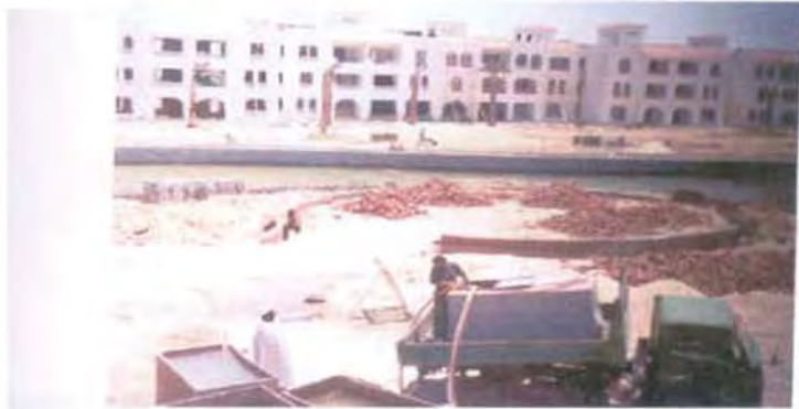
Fig. (7- 66) Bricks for building handling on site
