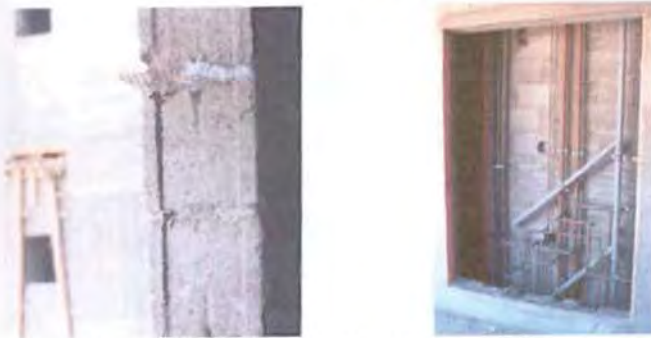
Fig. (7-45) Walls constructed according to specs, Fig. (7-46) Potable water pipes from copper
