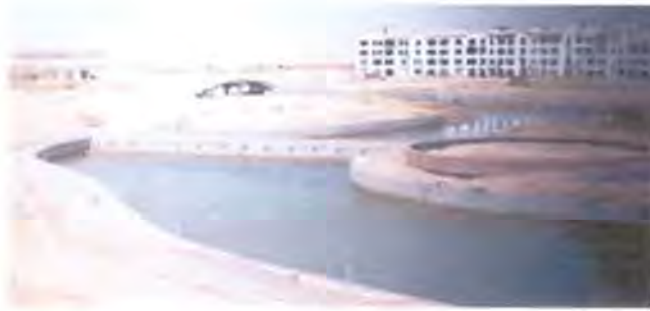
The view over looking the artificial lake Fig. (7-70)
