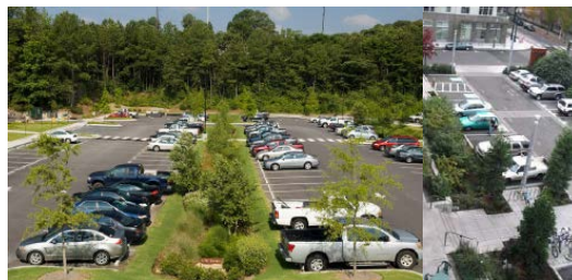
Fig. 5 Two methods of using bioswales in parking lots on the University of Regina Campus (DIALOG, 2011, p. 69)
