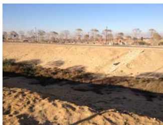
Fig. 7 One of the retention basins surrounding the parking areas
