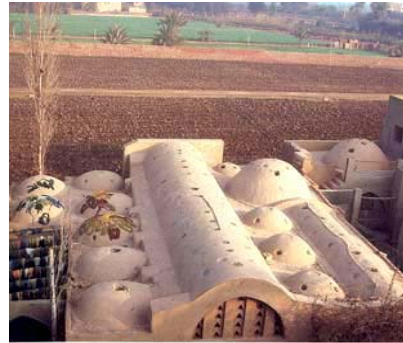
Fig (23): Oculi in the vaulting roof
