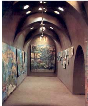
Fig (22): Daylight Shafts
