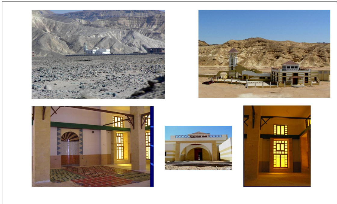
fig. 5. Abou Zenima Mountains of Sinai enclose the site of the project. The lines of the mountains match the mosque's strips. Numerous interior decisions were vernacularly participated by local laborers; source: authors,(2009)
