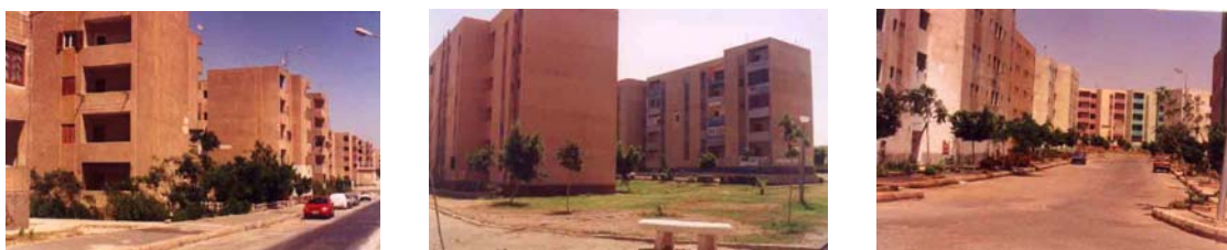
Figure 1: External features of the five story walk-ups.
