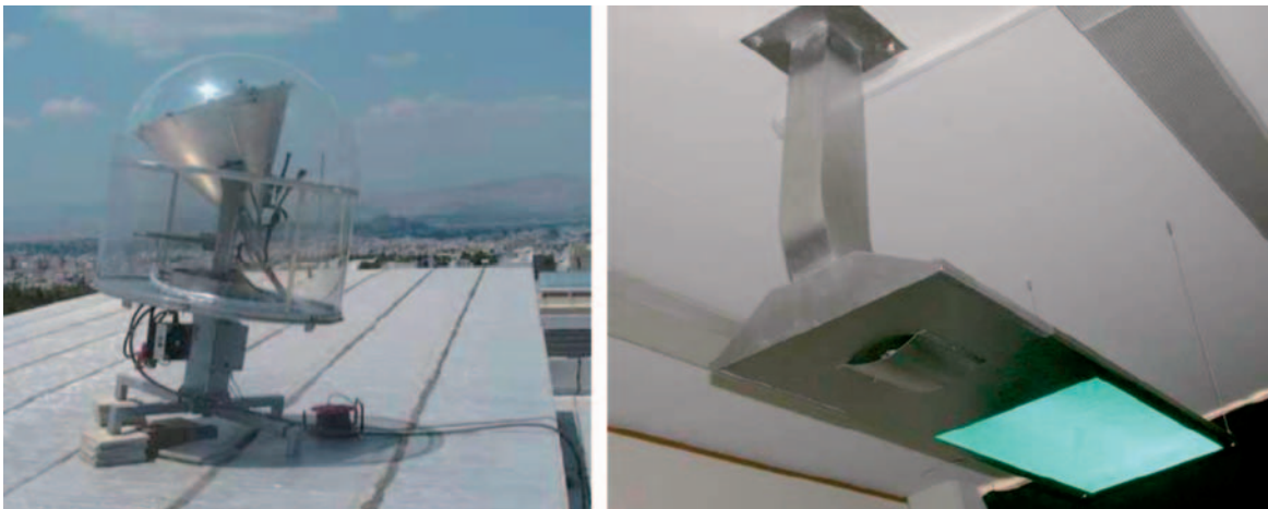
Figure 8 A universal fibre optics (UFO) collector and luminaire
