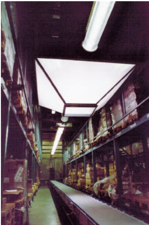
Figure 6 The Arthelio used to light a warehouse
