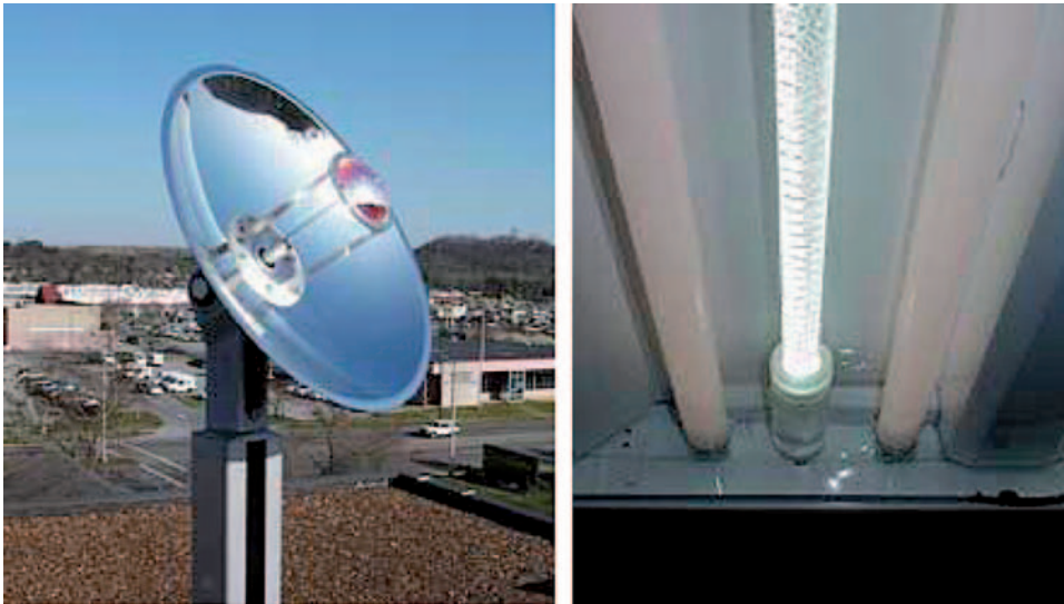
Figure 7 The hybrid solar lighting (HSL) collector and the hybrid luminaire
