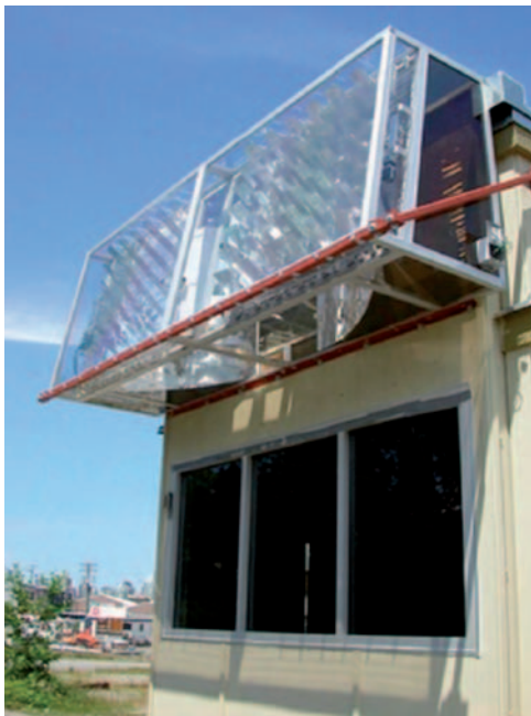
Figure 9 The solar canopy illumination system (SCIS) collector
