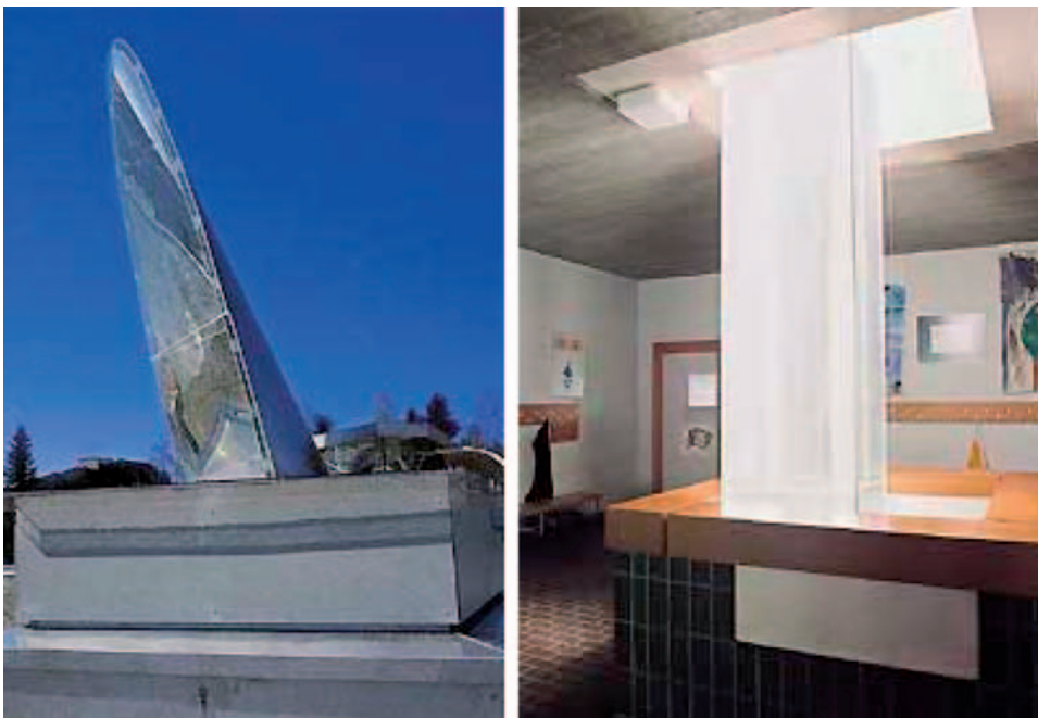
Figure 5 A Heliobus collector and the output device
