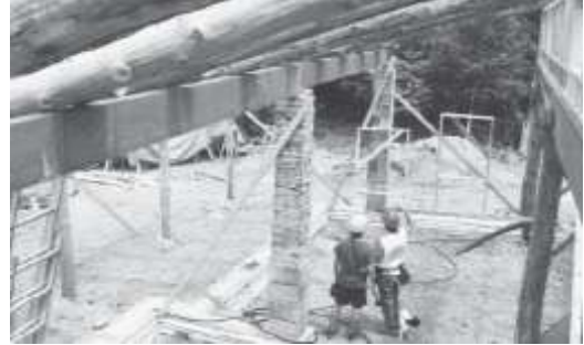
شكل 2- 8 أعمدة قطع الاخشاب Waste Wood Columns المصدر: Magwood, Chris, Building Better Buildings: A Comparative Guide to Sustainable Construction (Gabriola Island, Canada: New Society Publishers, 2014) (p. 62).
