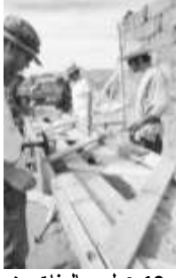
شكل 2- 10 عمل جمالونات من بقايا قطع الاخشاب المصدر: Kennedy, Pallets Joseph, Building Without Borders: Sustainable Construction for the Global Village (Ontario, Canada: New Society Publishers, 2004) (p. 64).
