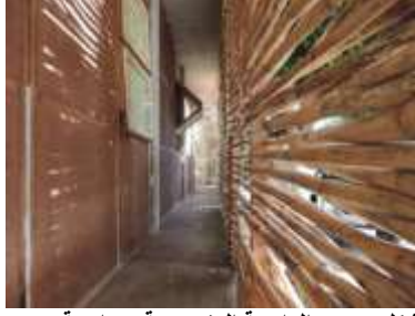
شكل 3- 44 الواجهة المزدوجة و واجهة البوص المكشوف بمبنى الاجتماعات المصدر: Pedro Bravo, 'In 4 Days, 100 Volunteers Used Mud and Reeds To Build This Community Center in Mexico', in Archdaily < http://www.archdaily.com/628163/in-4-days-100-volunteers-used-mud-and-reeds-to-build-this-community-center-in-mexico > [accessed 12 October 2015]
