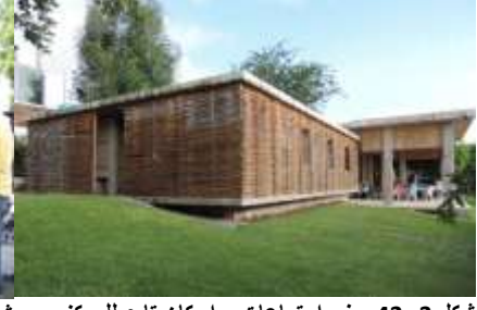
شكل 3- 42 مبنى اجتماعات و اسكان تابع للمركز المكسيكي للتنمية المحلية المصدر: Pedro Bravo, 'In 4 Days, 100 Volunteers Used Mud and Reeds To Build This Community Center in Mexico', in Archdaily < http://www.archdaily.com/628163/in-4-days-100-volunteers-used-mud-and-reeds-to-build-this-community-center-in-mexico > [accessed 12 October 2015]
