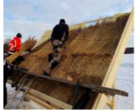
شكل 3- 50 تركيب السقف بنظام Thatch المصدر: Lautkankare, Rauli, 'The Fire Test of Thatched Roofs', in Guide Book of Reed Bussiness: Central Baltic Integration Program , ed. by Anne Hemmi (Estonia, Finland: European Regional Development Fund, 2013), pp. 32-37 (p. 1).
