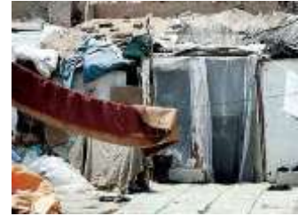
شكل 1- 1 البناء بالخرقة و البلاستيك بالهند المصدر: Taher, Mania T. and Ibrahim, Arafeen, 'Transformation of Slum and Squatter Settlements: A Way of Sustainable Living in Context of 21st Century Cities', American Journal of Civil Engineering and Architecture , 2 (2014), 70-76.
