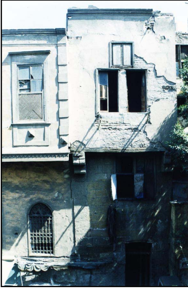
Figure 4-30 Façade overlooking al-Mahgar Street before rehabilitation (October 1998)
