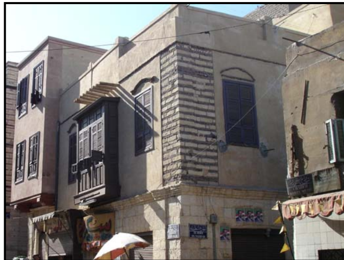
Figure 4-43 Bayt al-Khayātīn: Overview of the façade after intervention.
