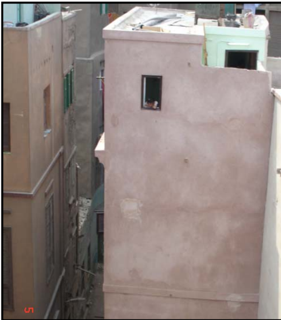
Figure 4-109 The wall after intervention (August 2005)
