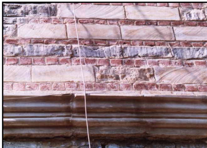
Figure 4-52 Façade after intervention (August 2004)
