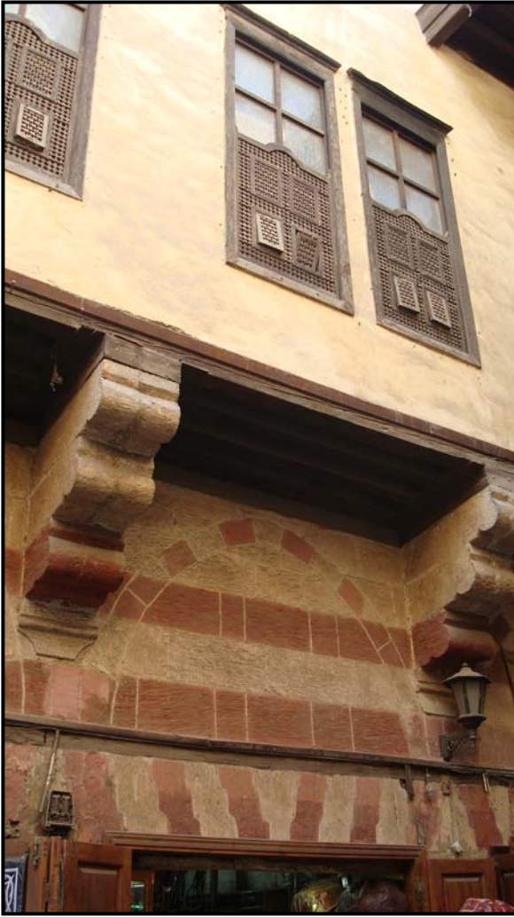
Figure 2-3 Residential units of qaṣabat Raḍwan bik in al-Darb al-Aḥmar, with stone corbels, Ablaq colored stone, and vertical sliding wood screen (18 th century)
