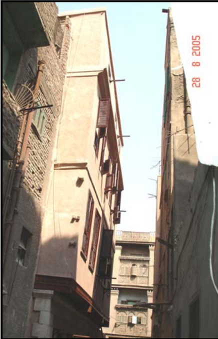
Figure 4-99 The Façade after intervention (August 2005)
