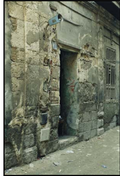
Figure 4-81 Entrance portal before intervention (February 2005)
