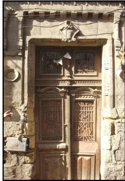
Figure 3-45 Entrance Portal of Bayt al-Ghandūr (February.2004)
