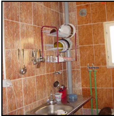
Figure 4-63 The kitchen after intervention (February 2005)
