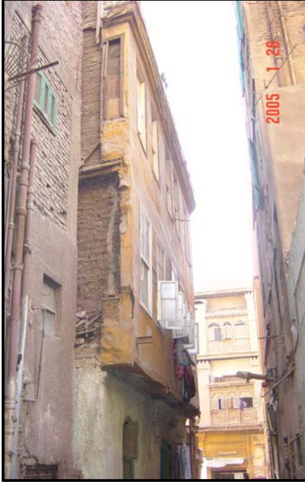
Figure 4-98 Façade overlooking Atfit al-Zila'i Looking east before intervention (January 2005)
