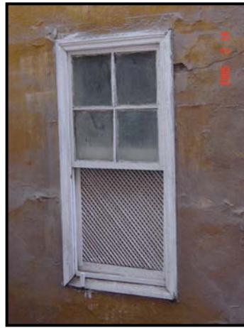
Figure 4-114 Window at the facade of the upper level before intervention (February 2005)
