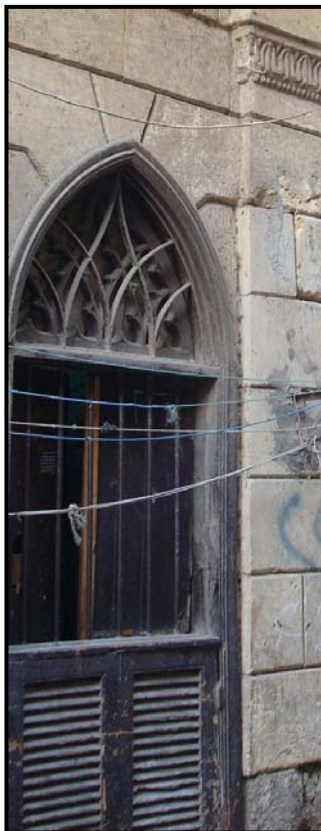
Figure 3-42 Pointed arch window of Bayt al-Najjarīn
