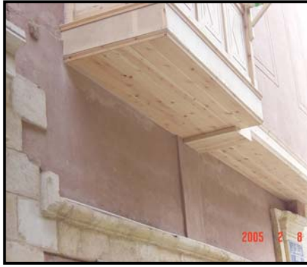
Figure 4-61 The southern façade after intervention (February 2005)
