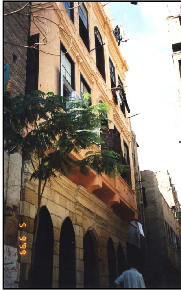
Figure 4-36 Bayt Al-Najjarīn after rehabilitation- façade overlooking al-Ḥara al-Nazifa (September 1999)
