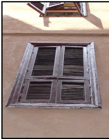
Figure 4-115 The window after intervention (August 2005)
