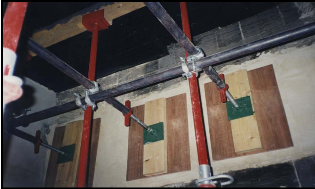
Figure 5-13 Metal horizontal shoring at Bayt al-Razzaz
