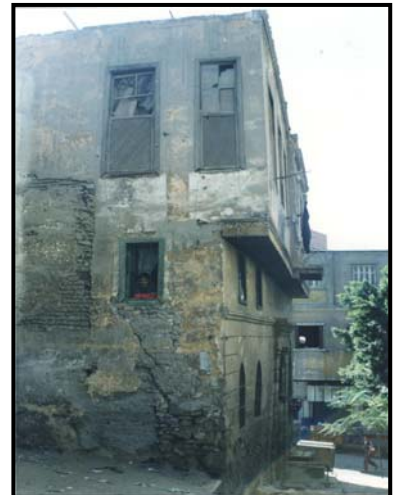
Figure 4-27 Disintegrating wall of Bayt Al-Sitt 'Awaṭif - East Façade before rehabilitation (October 1998)
