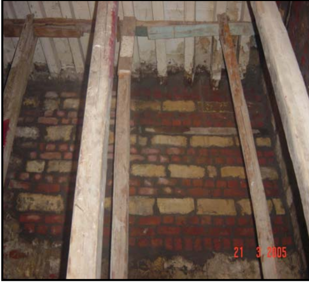
Figure 5-12 Shoring up the ceiling with wooden posts (March 2005)
