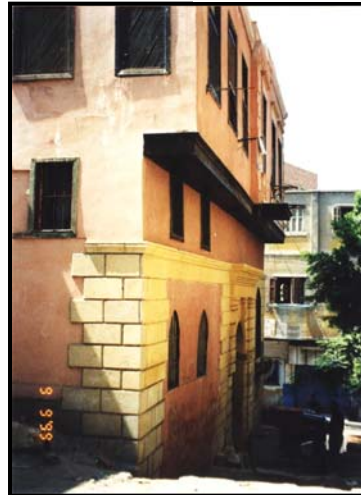
Figure 4-28 The Eastern façade after rehabilitation (September 1999)
