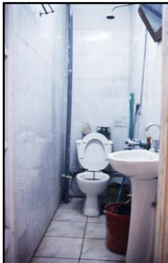
Figure 4-47 Floor paving of the first floor toilet -After intervention (September 2004)
