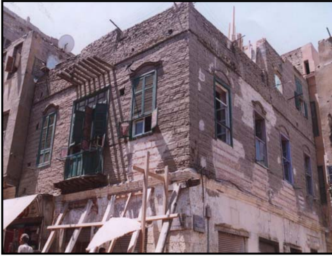
Figure 4-42 Bayt al-Khayātīn: Overview of the façade before intervention (August 2004)
