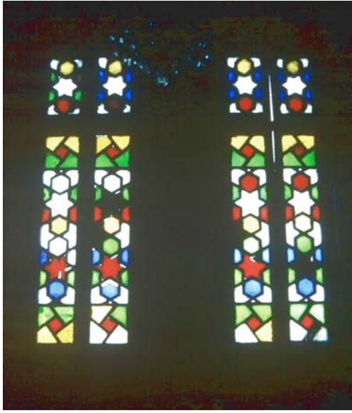
Figure 4-135 Internal view of the windows (May 2005)
