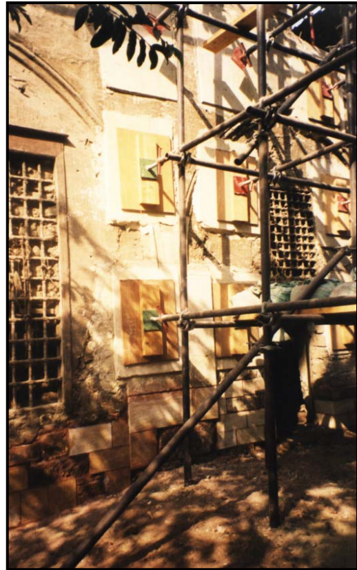
Figure 5-14 Metal horizontal shoring at Bayt al-Razzaz
