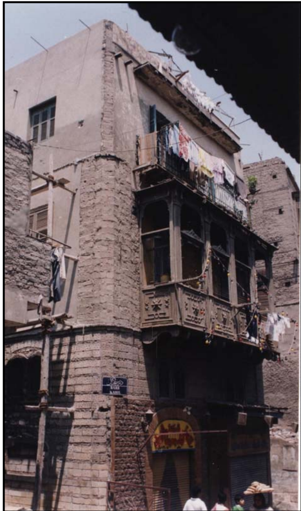
Figure 4-2 Overview of Bayt Sukkar before rehabilitation seen from al-Maḥgar Street (March 1998)
