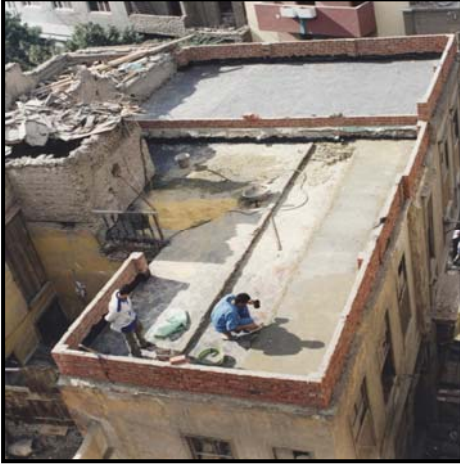
Figure 4-26 Bayt Al-Sitt 'Awaṭif during rehabilitation (September 1999)
