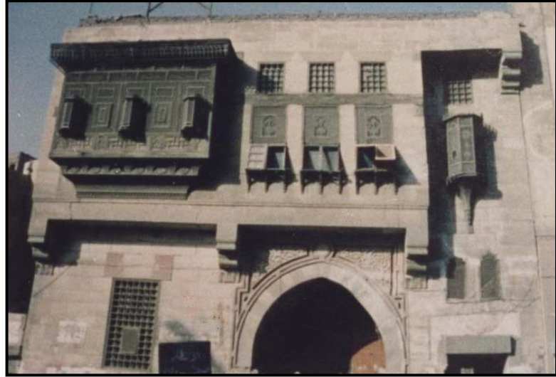
Figure 4-152 General view (May 2004)
