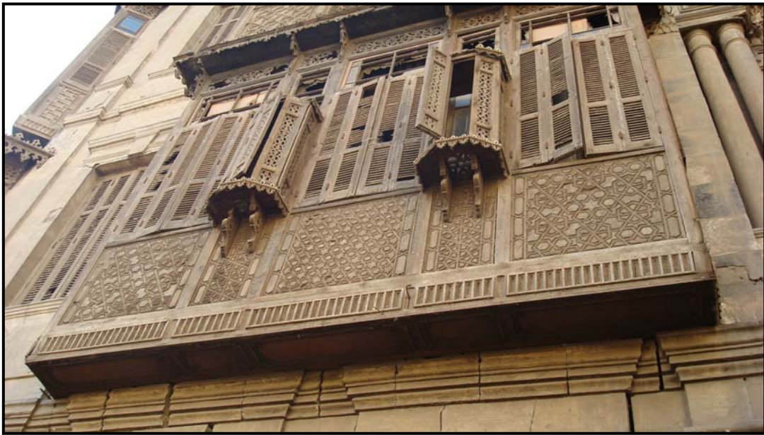
Figure 3-32 Bayt al-Qirabi wooden shutters decorative sill and projected booths for water jars
