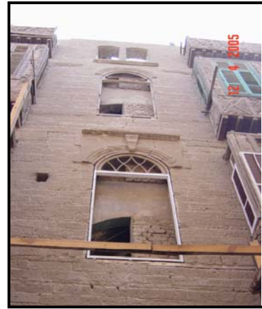
Figure 4-85 The central portion of the façade at the staircase before intervention (April 2005)
