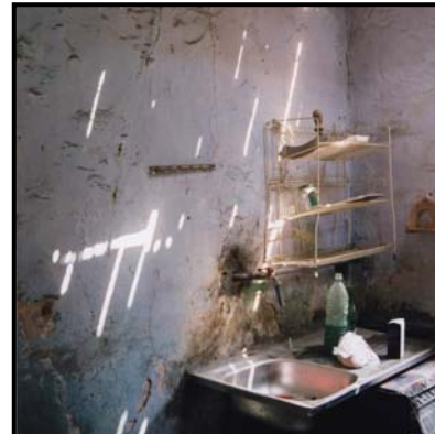
Figure 4-62 The second floor kitchen before intervention (November 2004)
