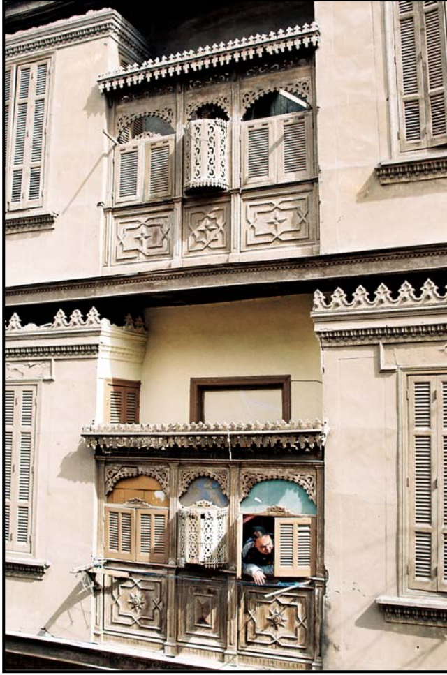
Figure 4-116 Façade of bayt Al-Ghandūr with typical mashrabiyya, note the separation between the floors in the cantilever. Photo credit: Walid al-Zunfali
