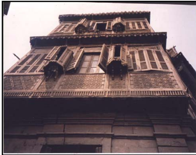
Figure 4-129 Street façade Bayt Al-Qirabi, showing the cylindrical mashrabiyya (May-2005)
