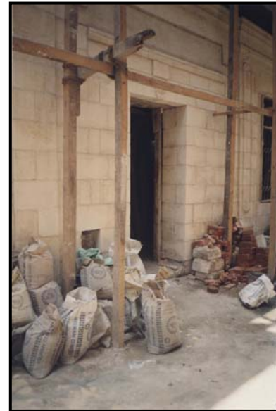
Figure 4-82 The entrance portal after replacing the deteriorated stones with new limestone blocks (August 2005)
