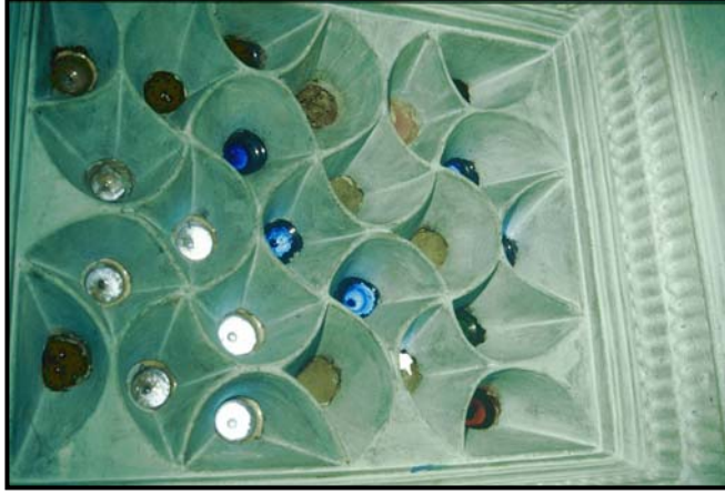
Figure 3-51 Qamariyya roof: The bathroom ceiling of Bayt al-Qirabi (May 2005)
