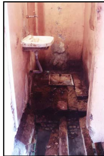
Figure 4-46 Existing condition of the Toilet of the eastern apartment (April 2004)
