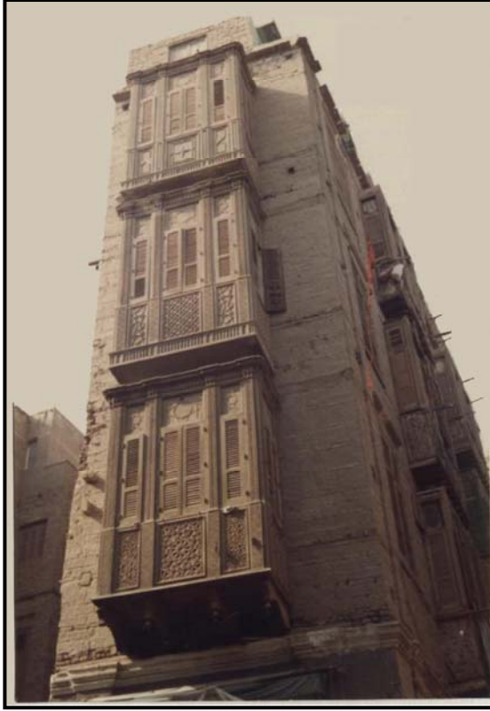
Figure 4-73 Bayt Abu al-Hasan seen from al-Mahgar Street before intervention (January 2005)
