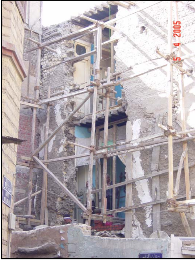
Figure 5-18 Vertical segment dismantled for reconstruction at Bayt Abu al-Hassan (April 2005)
