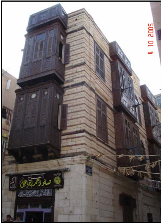
Figure 4-74 The mashrabiyya(s) of the facades after intervention (October 2005)
