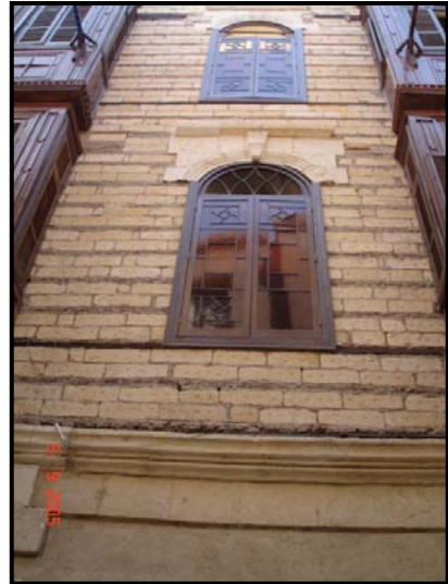
Figure 5-22 Stone façade in Bayt Abu al-Hasan after cleaning (September 2005)
