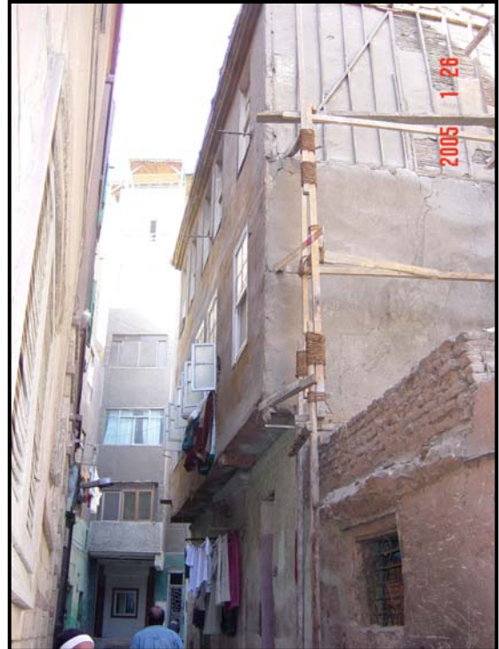
Figure 4-106 The façade before intervention (February 2005)
