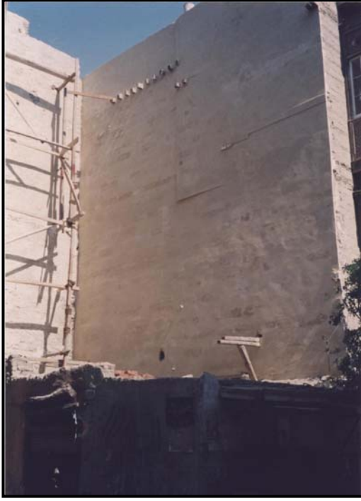
Figure 4-84 The southern façade after intervention (July 2005)
