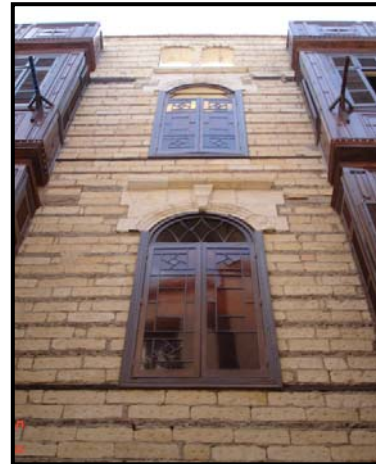
Figure 4-86 The Façade after cleaning the stones (September 2005)
