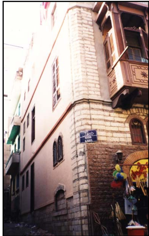
Figure 3-50 Facade cornices defining the floor levels in Bayt Sukkar.
