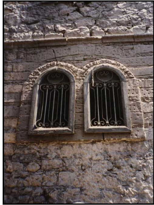
Figure 3-49 Stone Cornice in Bayt Sukkar
