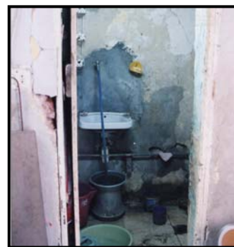
Figure 4-64 the bathroom of the second floor before intervention (November 2004)
