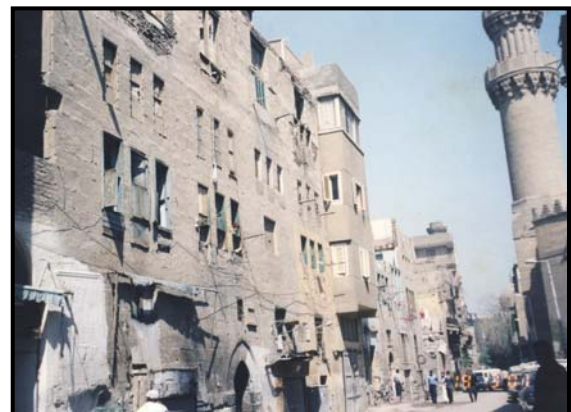
Figure 2-6 General view of Rab' Al-Tabbāna
