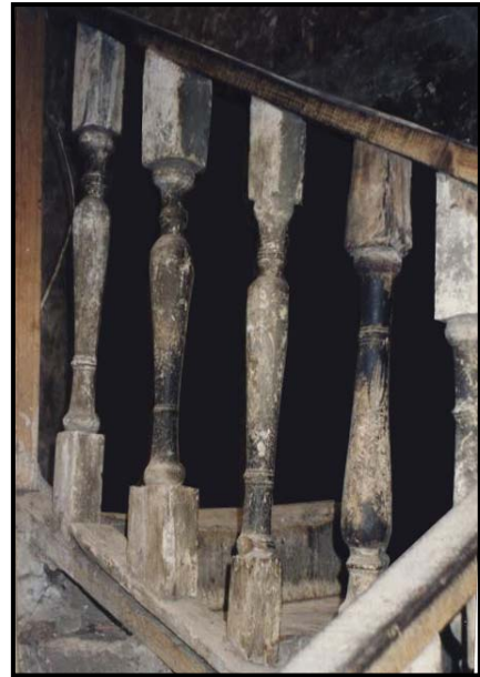
Figure 3-25 Typical Wooden handrail of 18th century in Bashtak house
