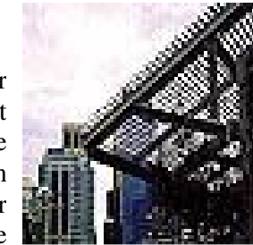
Fig(3-32) Louvers as external operable shading device www.squ1.com
