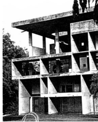
Fig.(1-39) Villa Shodhan Behling, Sophia & Stephen, "The Evolution of Solar Architecture" , p.176
