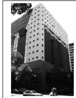
Fig.(4-5) Portland Building Utzinger, Michael and Wasley, James "Vital Signs, Building Balance Point" P. 19
