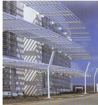
Fig.(3-22) Vice Chancellor's Office Jones, David Lloyd, " Architecture and the environment ", 1997
