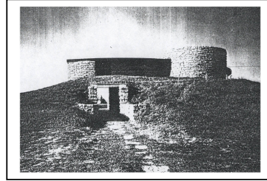
Fig.(1-42) The Solar Hemicycle- North Façade Pfeiffer, Bruce Brooks, "Frank Lloyd Wright" p.155
