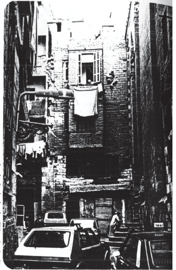
Fig. (60): Present condition
