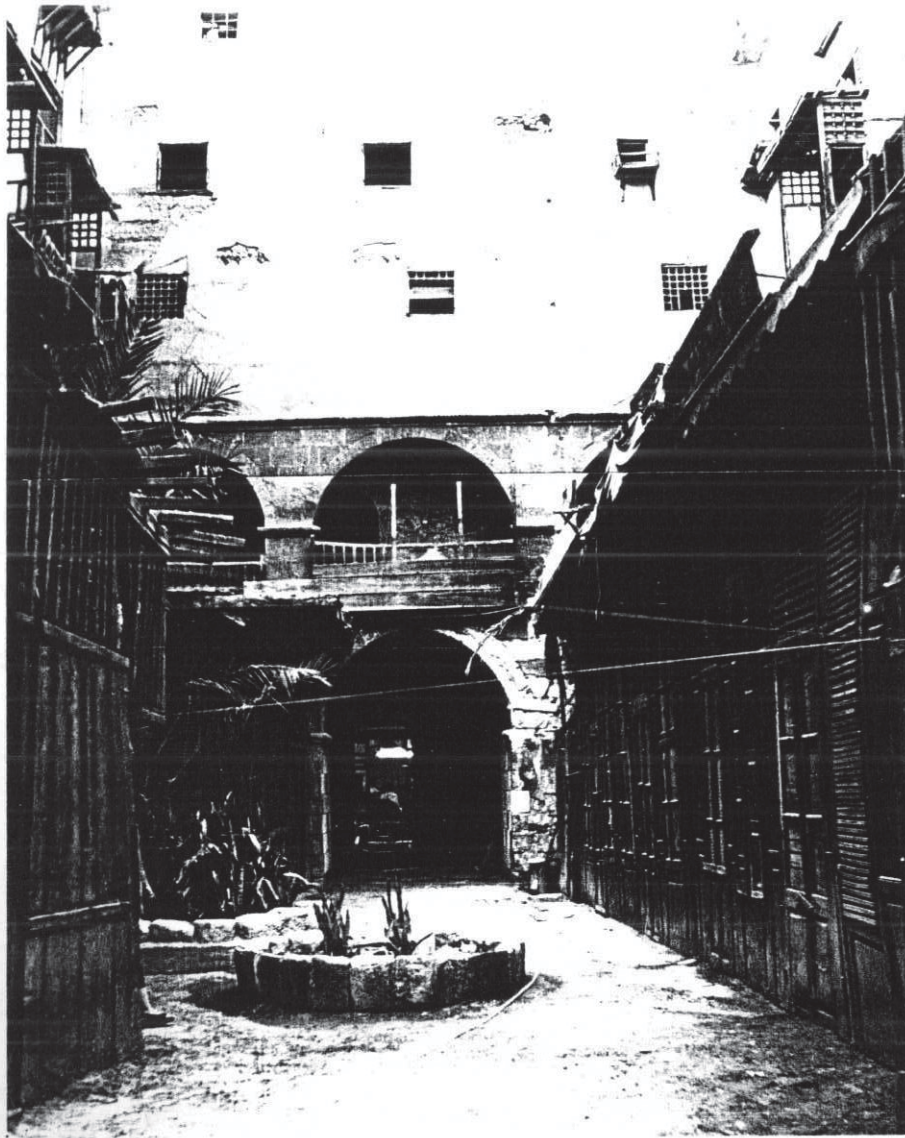
Fig. (9): Wakalat Bazaraa in Old Cairo, Egypt. The courtyard is almost full of wooden shelters built in it.
