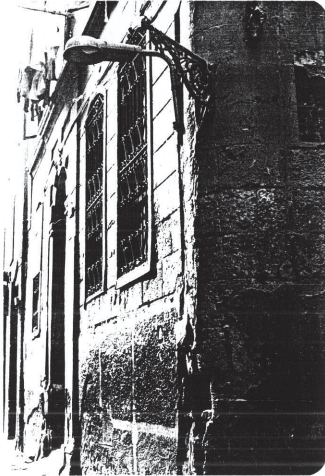
Fig. (64): Light installations which were once a piece of art were replaced by functional installations with no aesthetic value.
