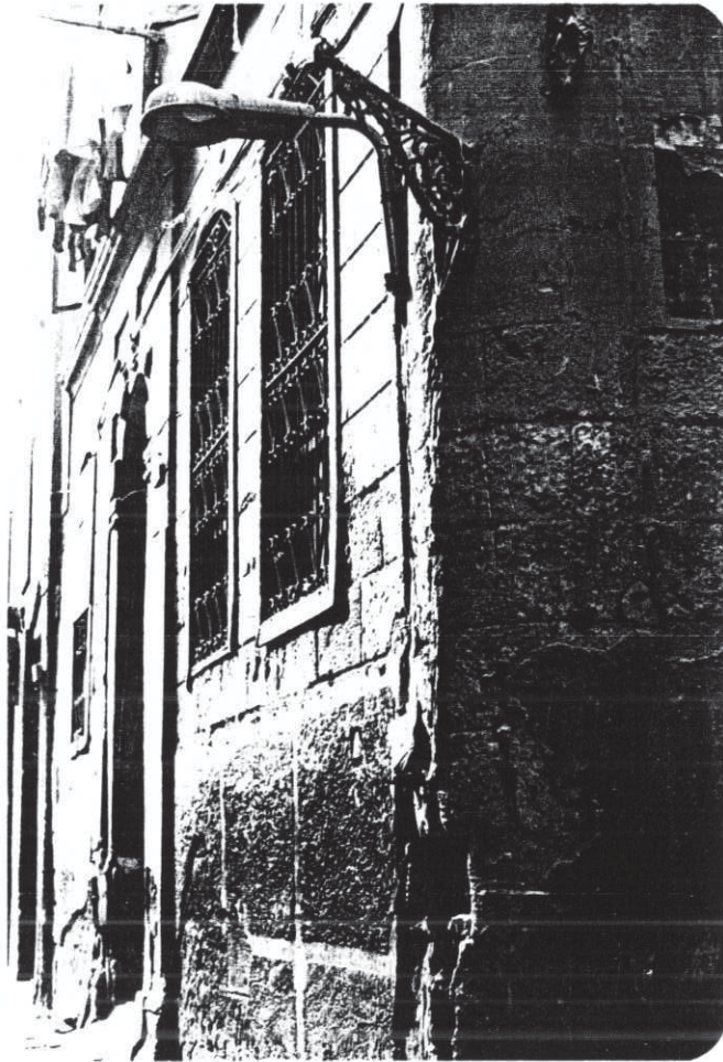
Fig. (64): Light installations which were once a piece of art were replaced by functional installations with no aesthetic value.
