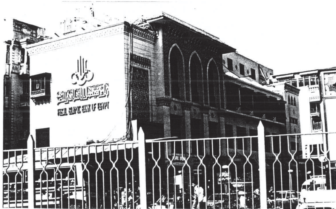
Fig. (8): A new concrete building keeping the character of the traditional architecture, Cairo, Egypt
