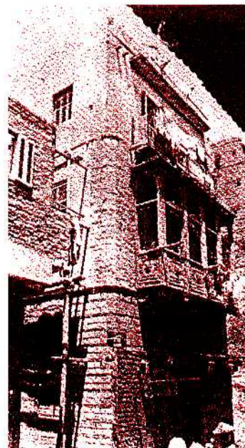
Bayt Sokkar before rehabilitation
