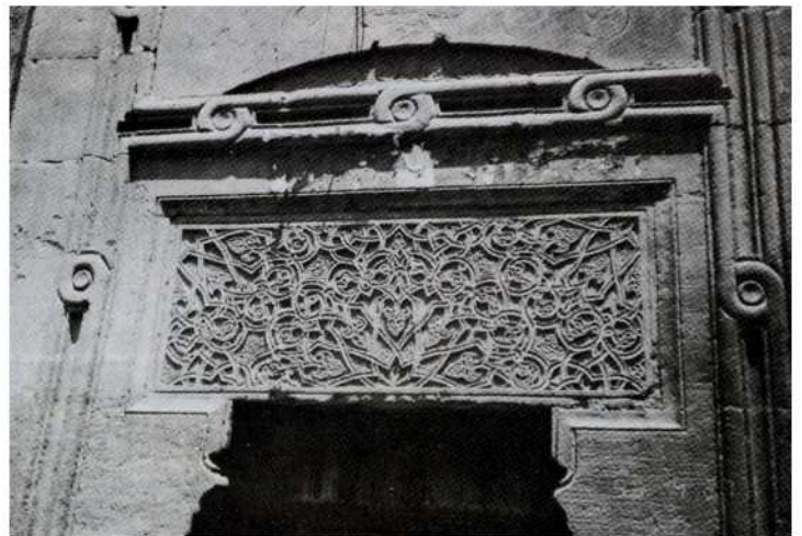
The Lintel above the Door to the Sabil
