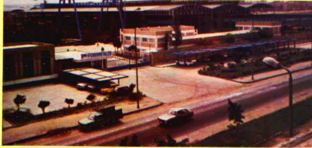
FERROMETALCO FACTORY - HELIOPOLIS - INDUSTRIAL ZONE
