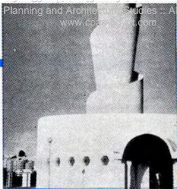
- A public lighting pole incorporating into a residential apartment building in Al-Khobar, Saudi Arabia.
