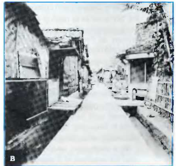
FIGURE 1A,B. Kampung improvement project, Indonesia: before and after. Source: R. Holod, ed., Architecture and Community: Building in the Islamic World Today (New York: Aga Khan Award for Architecture — an Aperture Book, 1983), p. 216.
