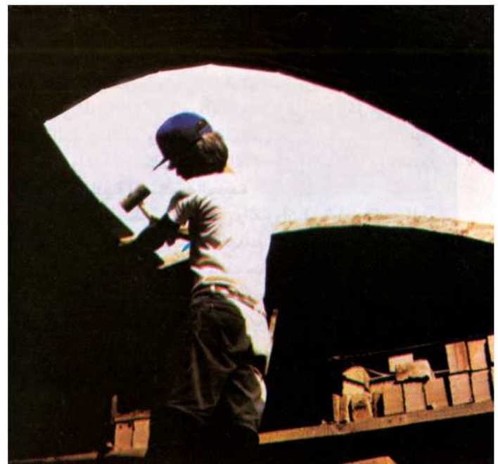
Fig. 8,9 : Construction of a mud brick dome without shuttering.
