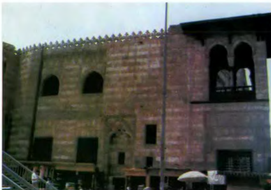
• Part of the facade on el-Azhar Street.
