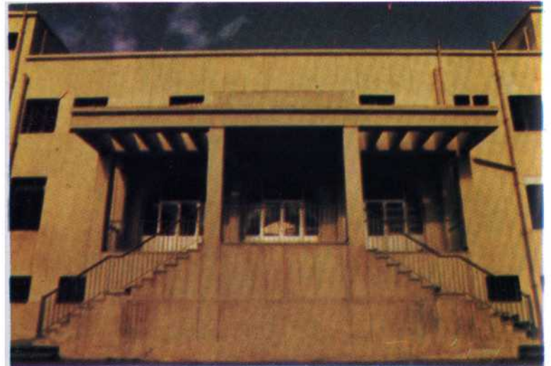
• The southern elevation.
