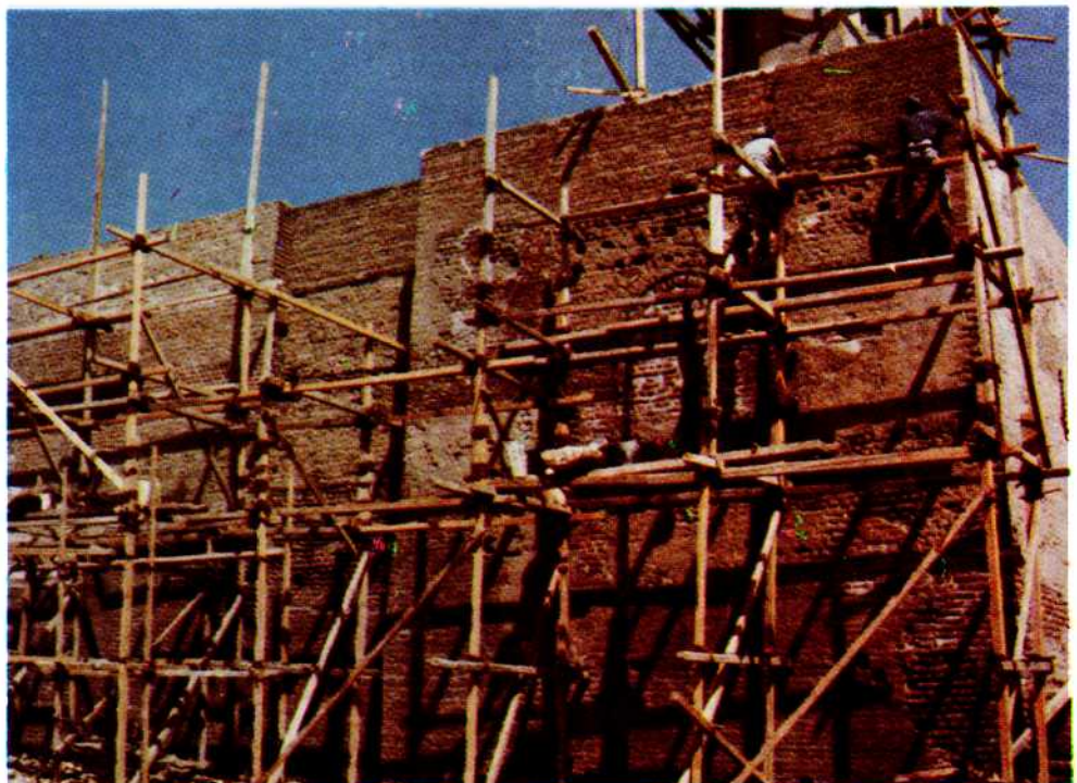
• Restoration work in the external facade of the Mosque.
