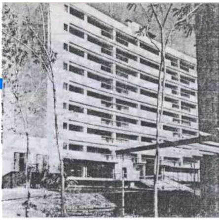
Nine-storey apartment building
