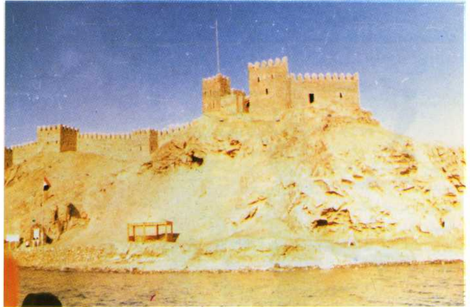
General view of the north fortification showing the facade of the bathroom, and the nourishment rooms in the central part, as well as the towers after restoration.
