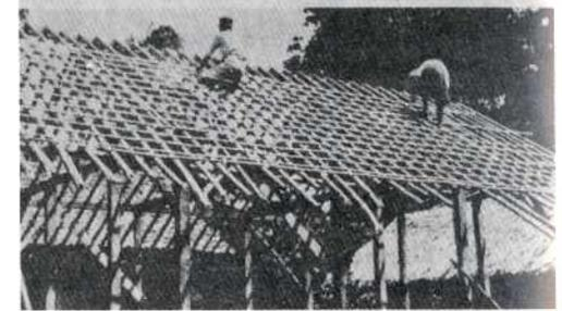
and notching, drastically reducing the strength of a bamboo culm, lashes are generally used as binding elements in framing. They may be split from the bamboo itself, or made from vines, reeds and bark of certain trees. Soft galvanized wire is also used for binding.
