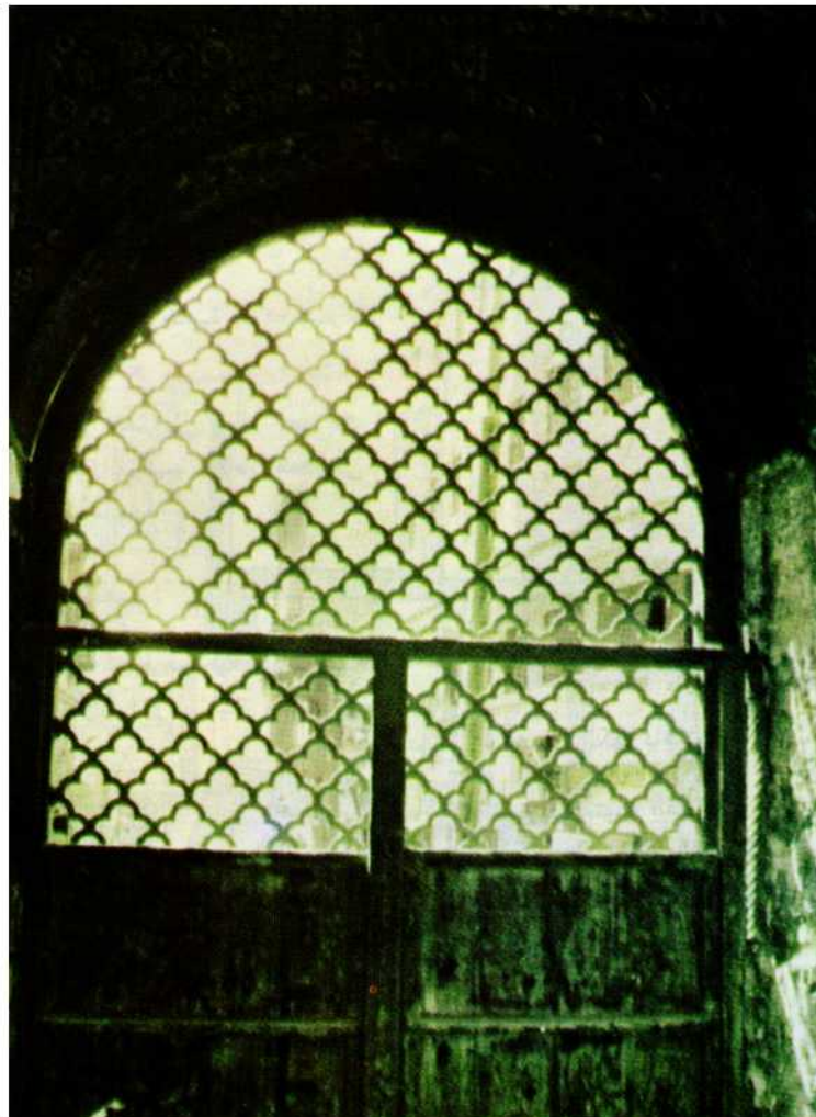
Bronze windows main elevation of the Sabil Kuttab (after restoration)
