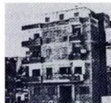
Example of Conventional Construction in Cairo
