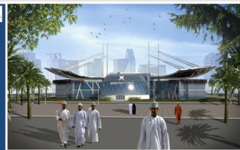
PERSPECTIVE SHOWING THE MAIN STRUCTURE SYSTEM MIXING BETWEEN TENT SYSTEM AND THE SPACETRUSSES
