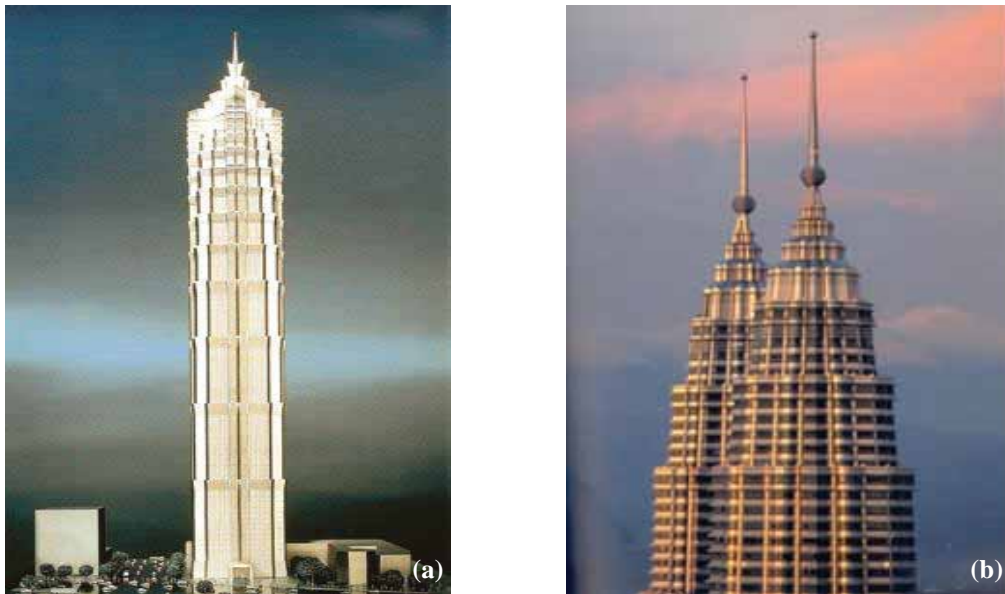
Figure (91) An example of Setback and sculptured tops, (a) Jin Maw Building, (b) Petronas Tower.
