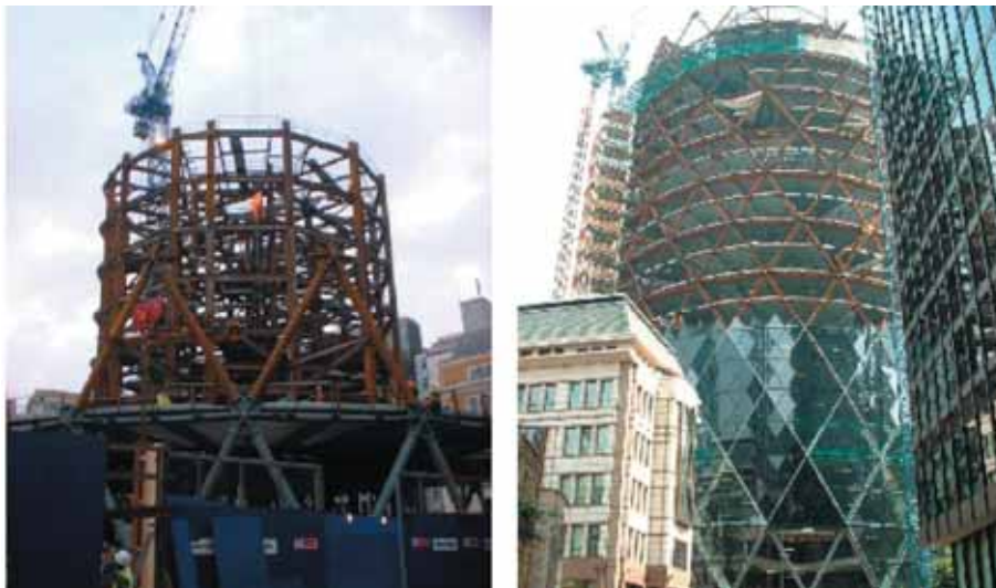
Figure (142) Construction process of Swiss Re building Ref: (Bridwell). P.113.
