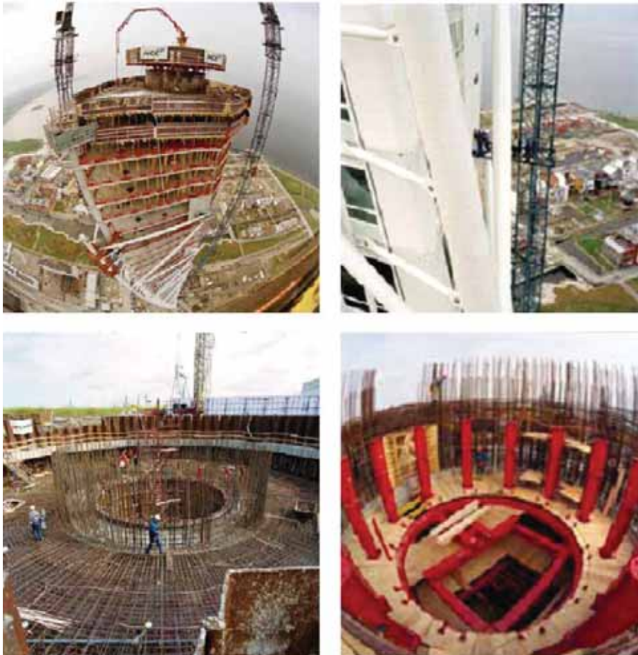
Figure (136) Construction process
