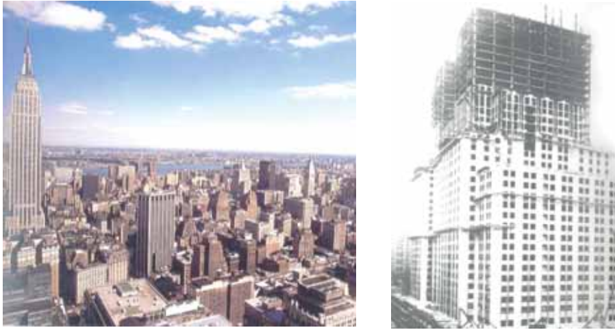
Figure (52) An Example of Using Shear Wall or Shear Truss Frame Interaction System, Empire State Building. Ref: (Ivan Zaknic 1998). P.200 & 201
