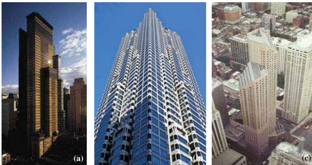
Figure (71) An example of using Concrete Bundled Tube System, (a) Carnegie Hall Tower, (b) One Peachtree Center (c) One Magnificent Mile building
