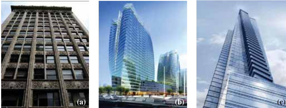
Figure (148) (a) Classical wall bearing expression although the system is not a bearing wall, (b) Modern curtain wall expression.
