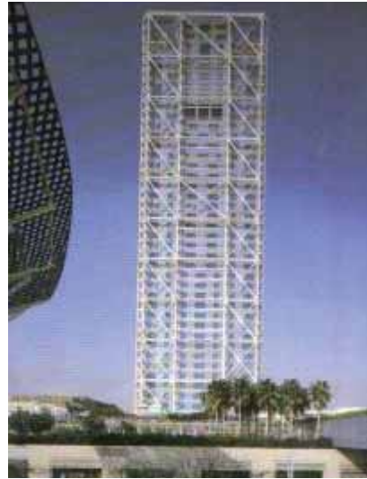
Figure (76) An example of using Exo-Skeleton System, (a) Hotel De Las Artes.
