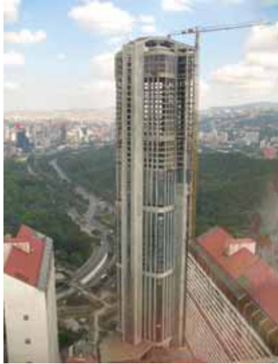
Figure (75) An example of using Super-Frame Structure System, (a) Parque central Tower.
