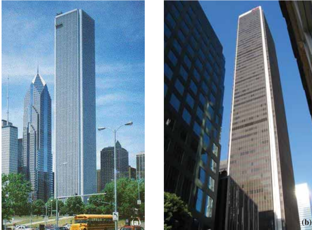
Figure (65) An example of using Framed Tube System, (a) Amoco Building, (b) AON Center.
