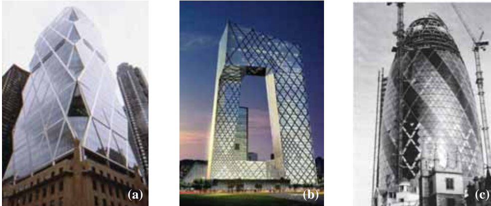
Figure (81) An example of using dia-grid structures in buildings' façade, (a) Hearst Tower, (b) CCTV Tower, (c) Swiss Tower.
