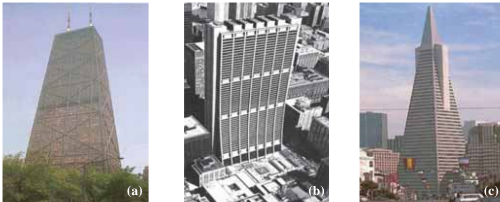
Figure (90) An examples of tapering effect utilization; (a) The John Hancock Center, (b) Chase Tower, The Transamerica Pyramid.
