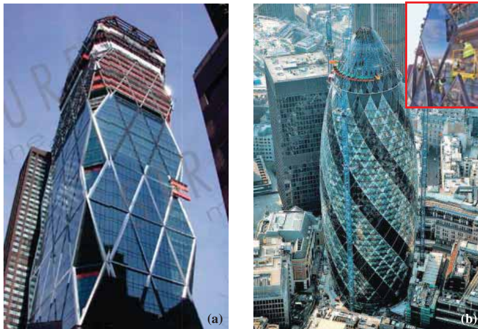
Figure (73) An example of using Dia-Grid Structure, (a) Hearst Tower, (b) Swiss re Building.
