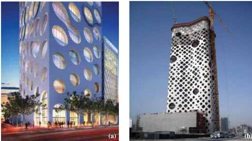
Figure (82) Another example of using diagrid structures in building's façade, (a) COR building, (b) 0-14building.
