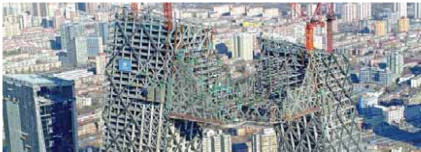
Figure (124) The Overhang before connection
