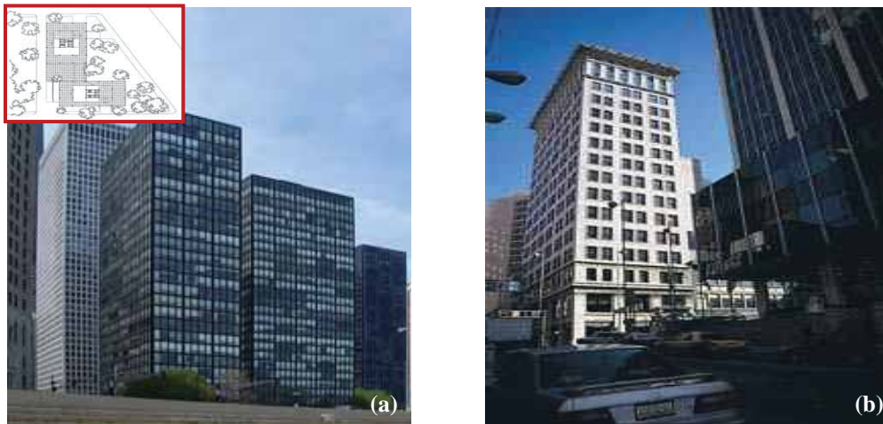
Figure (42) An example of using Moment resisting frame. (a) 860 & 880 Lake Shore Drive Apartments, (b) Ngalls Building.
