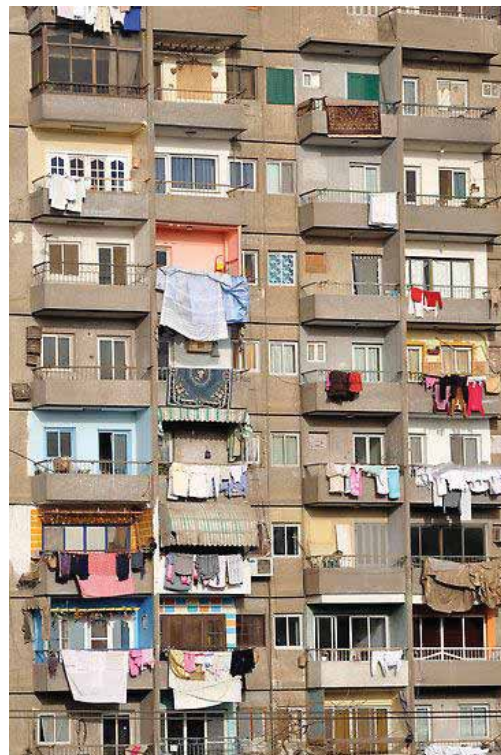
Figure 3.21: Balconies of Apartment Block in Cairo
