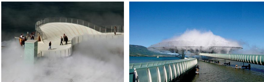
(Fig. 4.4-4.5) the mist is the main theme of the building creating a new experience to the users
