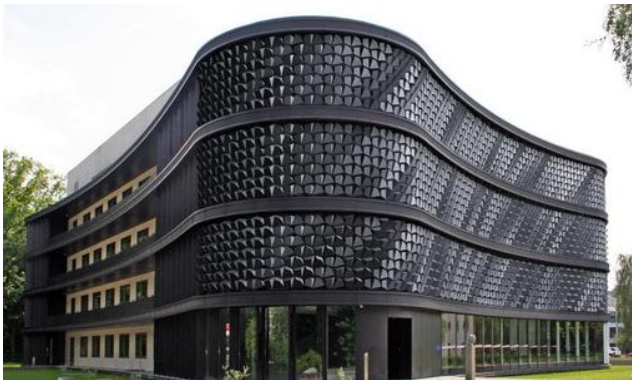
(Fig.4.24 ) The flare installed on a mock up building in berlin originally designed by Staab architects making the building more interactive to their surrounding environment
