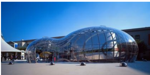
(Fig 3.6): Bernhard Franken's BMW pavilion in Berlin that was formed from individual glazing panels curving in a three dimensional curve to cause a dramatic effect.
