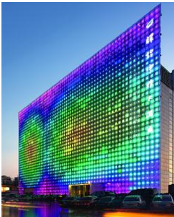
(Fig. 4.20) The GreenPix Zero Energy Media Wall makes the Xicui entertainment complex in Beijing an artistic medium with a social conscience, using photovoltaics to generate energy.
