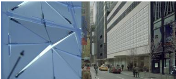
(Fig. 3.3): Pixel skin is developed as a modular surface made up of robotic pixel tiles. Each panel has 255 potential states of adjustment, in order to create moving patterns and imagery. 13
