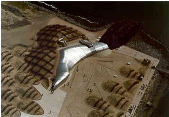
(Fig. 4.1) water pavilion layout and the two pavilions salt water and fresh water with its non-Euclidian form shaped as a sculpture. The pavilion has evolved from a three-dimensional computer model.
