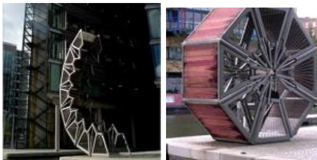
(Fig. 1.28): Rolling bridge, England.
