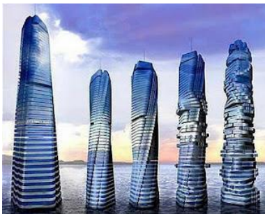
(Fig. 4.48) The 'tower in motion' - the world's first such building - is a revolutionary project based on Dynamic Architecture, creating unrepeated shapes
