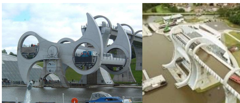
(Fig. 1.21): Falkirk Wheel Scotland, movable structure
