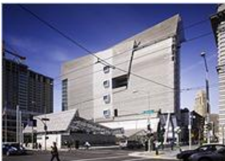
(Fig. 4.9)The new San Francisco Federal Building, designed by Thom Mayne: The exterior includes a screen that curls just over the top of the building.
