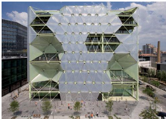
(Fig. 4.29) The Media-TIC façades are made of the eco-efficient material ethylene tetrafluoroethylene (ETFE) cladding.
