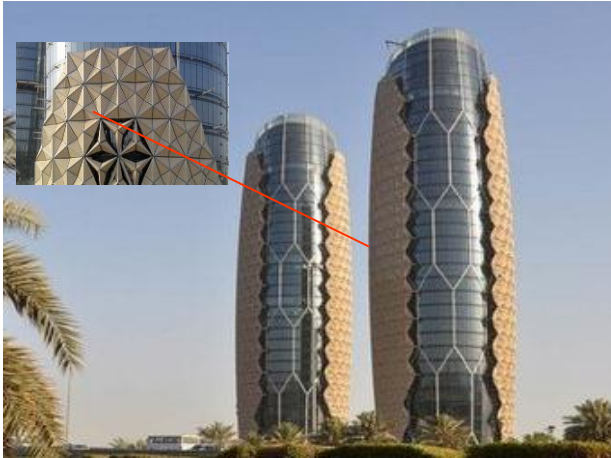
(Fig. 1.29): Al “bahar” tower in Abu Dhabi. The façade of triangular prototype is computer-controlled to respond to optimal solar and light conditions. Each triangle is coated with fiberglass and programmed to respond to the movement of the sun as a way to reduce solar gain and glare.
