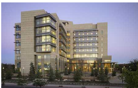
(Fig. 3.56)- United States Courthouse, Fresno, California, A system of distinctive precast concrete wall panels form an irregular pattern of folds, extrusions and corrugations across the building’s buff-colored surface.
