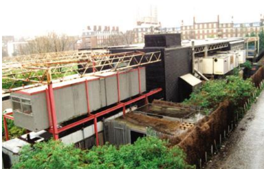
(Fig.1.6): Cedric Price, the “Inter-Action Centre”, 1977. The framework structure with plug-in, readymade port cabins used for offices, toilet rooms, and utility spaces.
