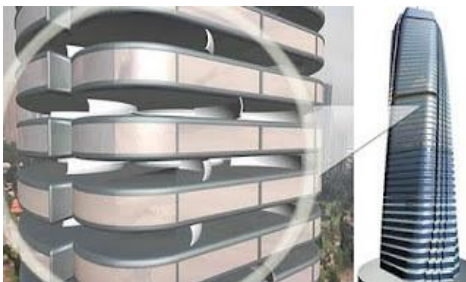
(Fig. 4.49) the turbines located between each floor and the photovoltaic cells on each roof
