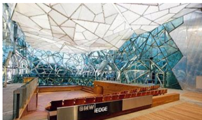
(Fig. 3.10): The atrium utilizing a limited number of standard components. A series of non-uniform frame shapes have been developed to form a continuous structure. The lattice supports glass panels on both its inner and outer faces.
