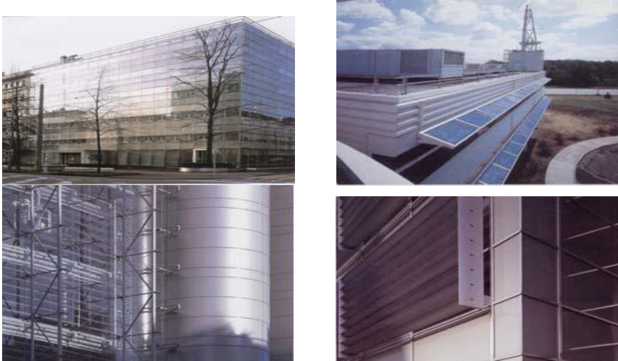
Figure 2-5 the Building Envelope as a communication interface, and feature of expressionism for environmental sensibility and technological sophistication: SUVA Building, Basel; Combined Brise-Soleils and PV panels; and Movable parts in the Helicon, Lond. And Microelectronics Buildings, Duisburg (Source: Lloyd Jones, David, "Architecture and the Environment: Bioclimatic Building Design". The Overlook Press, New York (1998) p 206).
