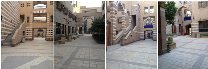
Fig. 173 Very similar different internal courtyards of HUSS
