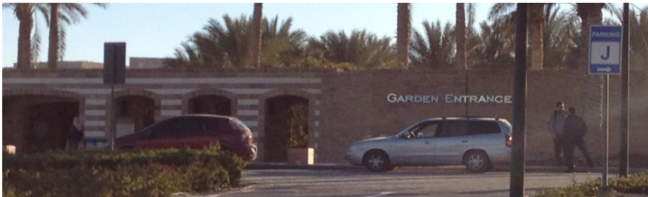
Fig. 135 One of the pedestrian gates attached to the main garden
