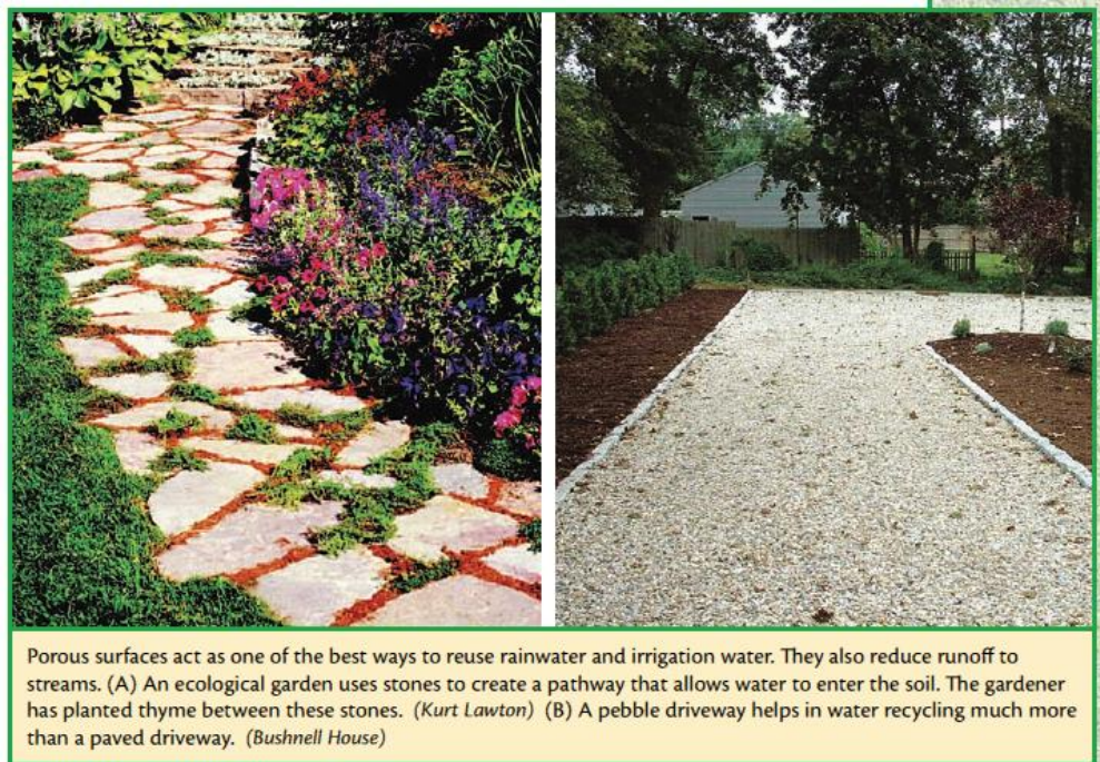
Fig. 23 Different designs of porous pavements (Mackzulak, 2010, p. 152)
