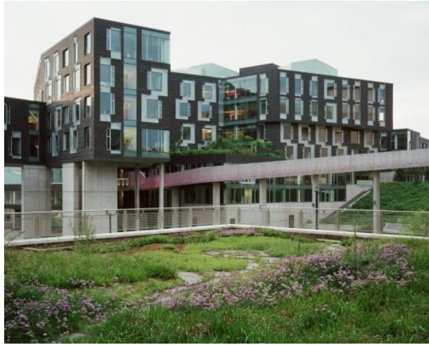
Fig. 28 Photo of Doherty Hall and Gates Center green roofs courtesy of Brad Temkin, 2011 (Carnegie Mellon University, 2014)
