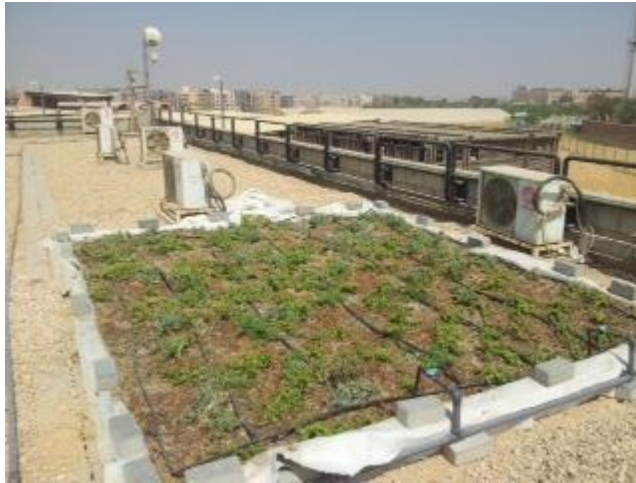
Fig. 157 Green roof for vegetables over RISE building
