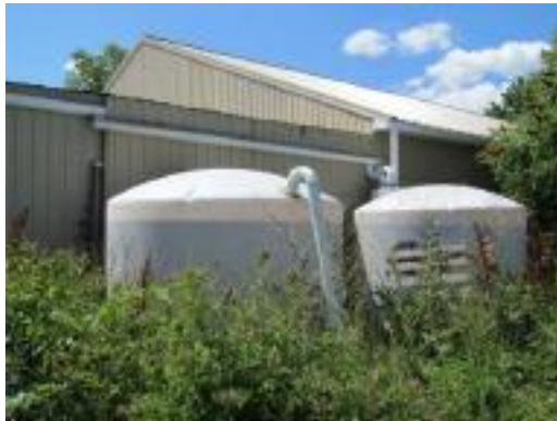
Fig. 22 A side view of the Horticulture Services Building (Macdonald Campus, Sainte-Anne-de-Bellevue, QC, Canada) (Adamowski, 2014)
