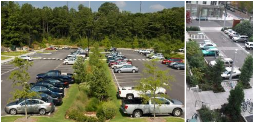
Fig. 31 Two methods of using bioswales in parking lots on the University of Regina Campus (DIALOG, 2011, p. 69)
