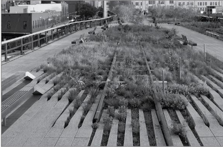
Fig. 50 The existing rail structure of The Highline that was reused as a neighborhood park and promenade (Calkins, 2012 kindle version, p. 8454)
