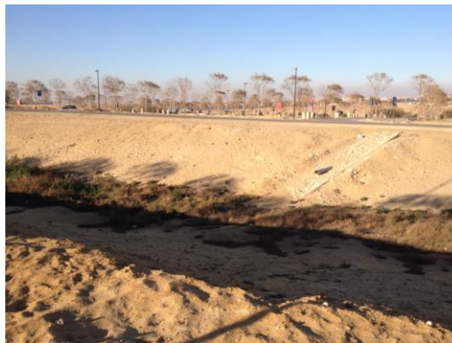
Fig. 155 One of the retention basins surrounding the parking areas
