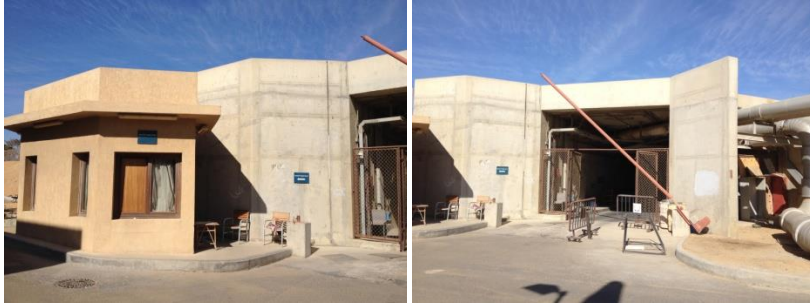
Fig. 138 The entrance of the underground tunnel
