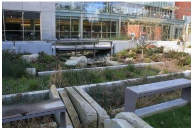
Fig. 25 Rain garden on the University of Seattle Campus (Seattle University Campus, 2014)
