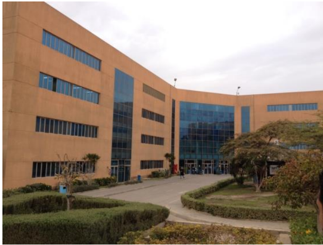
Fig. 121 The façade design of most GUC buildings
