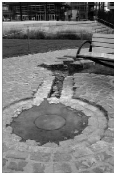
Fig. 19 The recirculating rain water system at Tanner Springs Park in Portland, OR, is an excellent of water that is safe and touchable because of the small shallow design (Calkins, 2012 kindle version, p. 2633)
