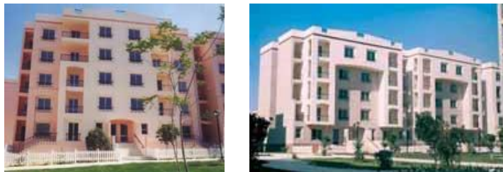
Figure (5.39): Example of high Albedo buildings' colors within Al Rehab City Source: (Al Rehab City, 2011)
