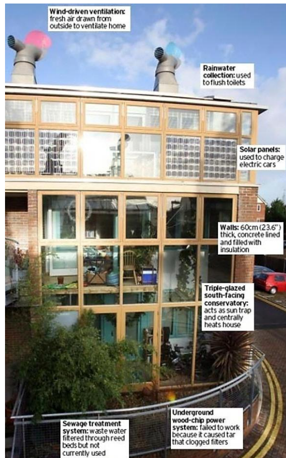
Figure (4.14): The integrated PV panels used in BedZED's buildings Source: (Telegraph Media Group, 2013)
