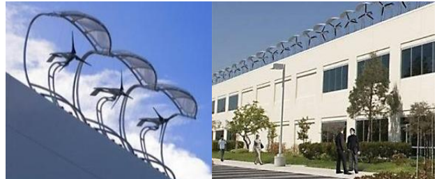
Figure (3.102): Example of the mini wind turbines used at buildings Source: (Chino, 2008)
