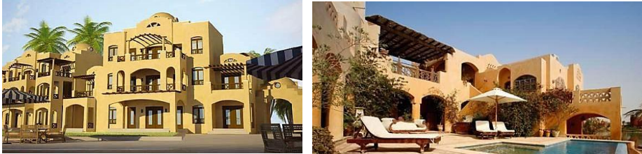
Figure (4.73): Shows examples of El Gouna buildings which used different shading elements Source: (Prime living, 2013)
