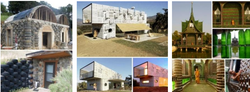
Figure (2.32): Example of recycling materials like: tires, wood pallet, bottles Source: (WebEcoist-Going Beyond Green, 2014)
