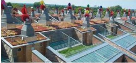
Figure (4.12): Roof lights used in BedZED Source: (Lazarus, 2002)
