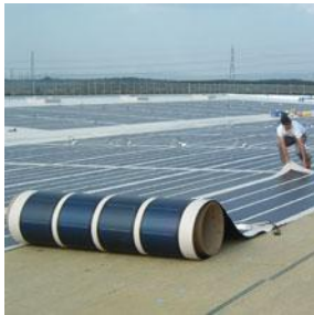
Figure (3.97): New flexible solar modules Source: (Energies-Renouvelables, 2012)
