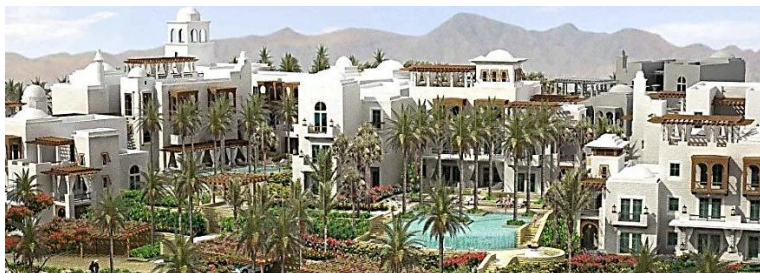
Figure (4.72): Shows examples of the window shapes in Ancient Sands Golf Resort Source: (Ancient Sands Golf Resort, 2009)
