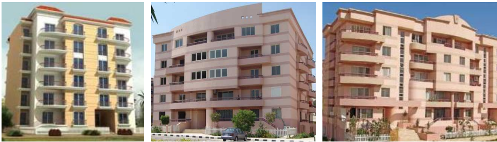
Figure (5.42) Lack of shading devices at the buildings' elevation in Al Rehab City Source: (Al Rehab City, 2011)
