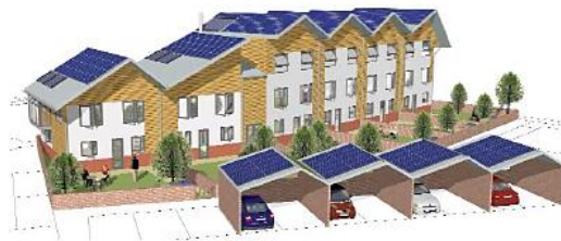
Figure (3.96): Pv on parking lots at BedZED Source: (Lazarus, 2002)
