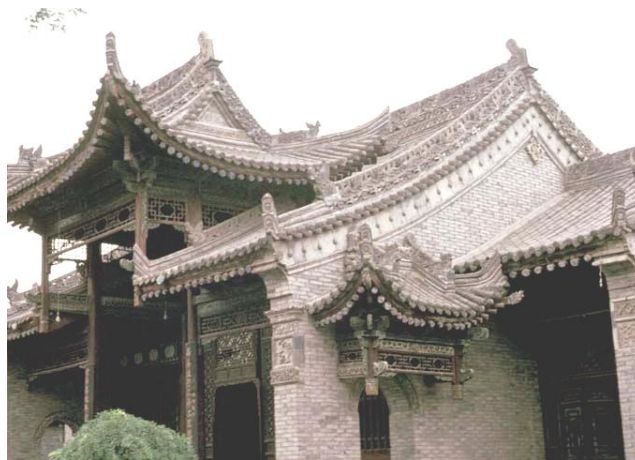
Fig. (1.11): A Detail of the upswept roof eaves at the Unmatched Pavilion of the Great Mosque, Xian, China. (Source: Archnet.org)
