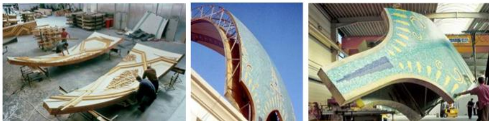
Fig. (3.111): Shots showing the installation process of goktepe mosque dome.
