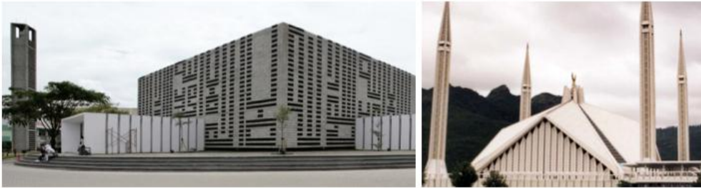
Fig. (3.105): Exterior views showing the forms of Irsyad and Islamabad mosques.
