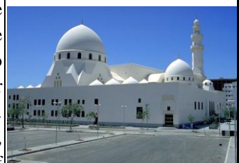
Fig. (3.52): Exterior view of the eastern façade. (Source: Archnet.org)
