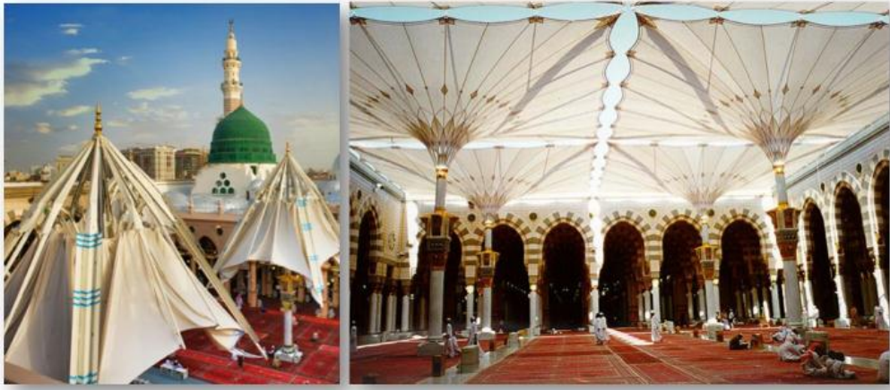
Fig. (3.109): Mechanically operated Teflon umbrellas used in the inner courtyard of the Prophet's Mosque.
