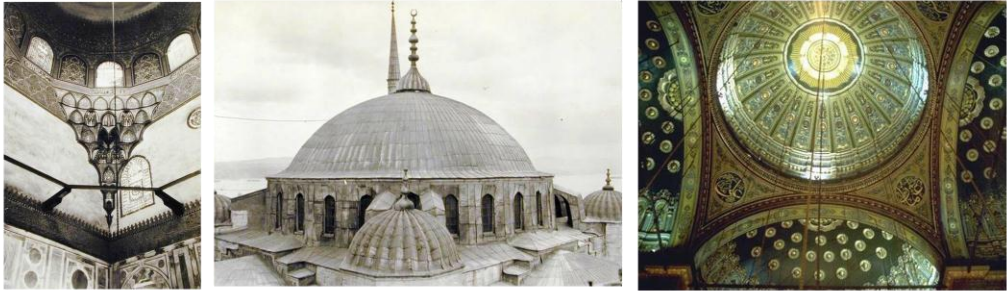
Fig. (1.27): The pendentives carrying the dome of the sultan barquq mosque, Cairo, Egypt (1398-1411 A.D.), the central dome of the ottoman mosques suitably highlighted by the diminutive scale of the surrounding ones of Sultan Ahmet mosque, Istanbul, turkey (1607-17 A.D.), and in Muhammed Ali mosque, Cairo, Egypt (1828-48 A.D.) (Source: Archnet.org), respectively.
