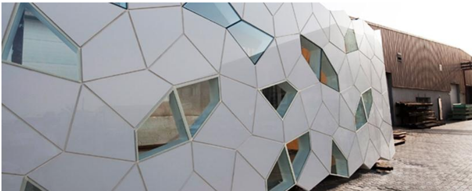
Fig. (2.23): Façade of Rak gateway, Ras Al Khaimah, Emirates. (Source: http://www.pct.ae/composite_projects.php?project=18 )
