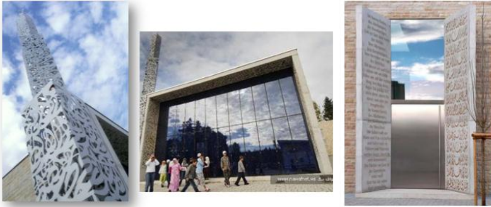
Fig. (3.103): Exterior view of the mosque, showing steel calligraphy used in the minaret, glass wall, and entrance concrete slabs of glass mosque.
