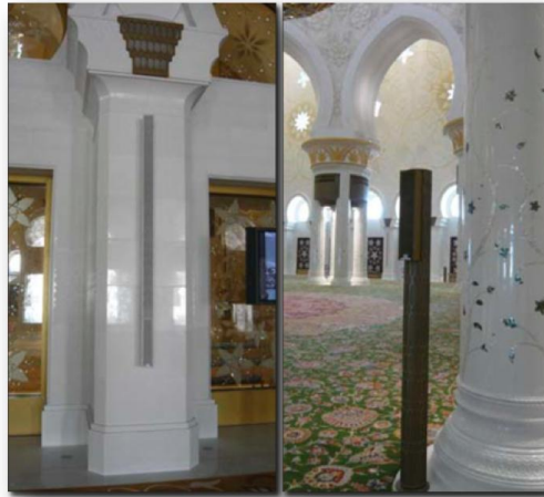
Fig. (3.113): The loudspeakers located inside the prayer hall of al sheikh zayed mosque.
