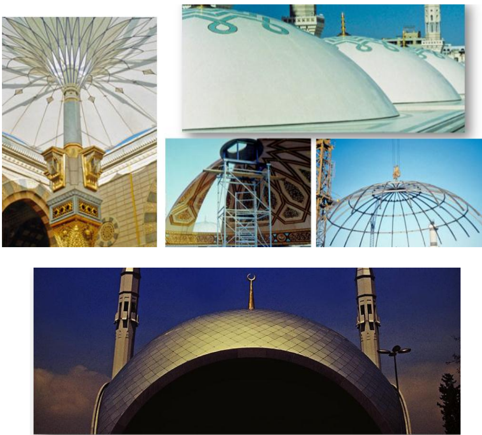
Fig. (3.97): Steel frames, teflon umbrellas, composites materials, and aluminum composite panels used in Prophet's, and Sakirin Mosques, respectively.
