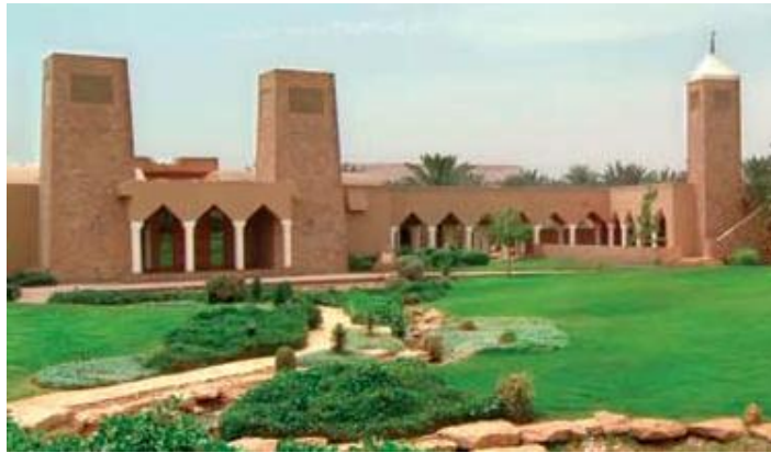
Fig. (2.17): Wind Towers in Al-Ruhmaniah Mosque, Saudi Arabia (Source: http://alrahmaniah.org/en/design/design.html )
