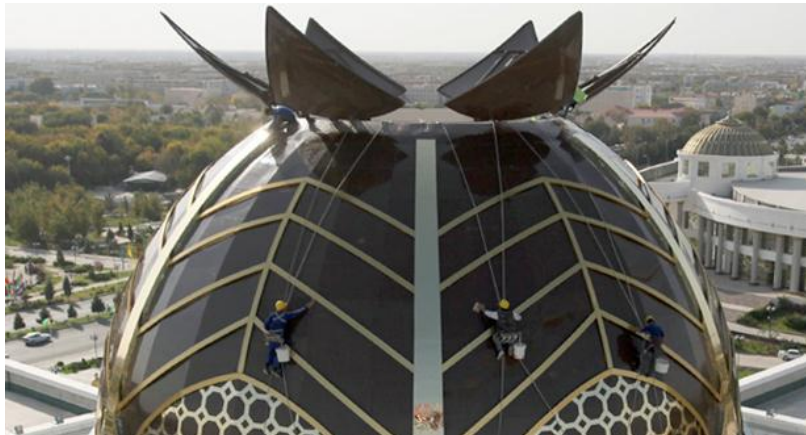
Fig. (2.24): Exterior view of Astelco Telescope Dome in Turkmenistan. (Source: http://www.pct.ae/composite_projects.php?project=25 )
