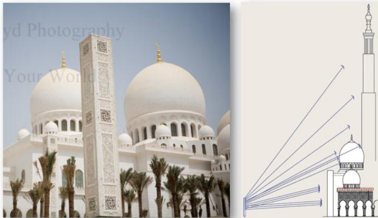
Fig. (3.102): Exterior view of the mosque, showing the projectors towers located around the building.
