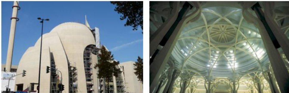
Fig. (3.106): Exterior view of cologne mosque, and interior view of the arches and ribs inside the prayer hall of Rome mosque, respectively.
