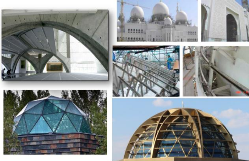
Fig. (3.98): Cast concrete, stainless steel structures, ribbed steel dome, materials used in Assyafah, sheikh zayed, glass dome mosque and sami ali pasha mosques, respectively.
