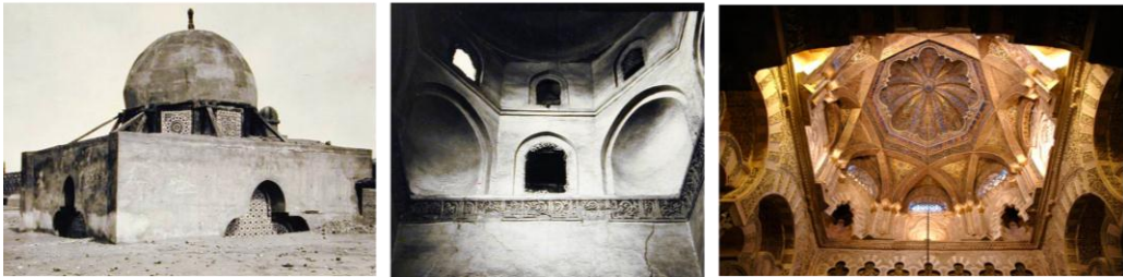
Fig. (1.26): The dome over the mihrab bay of Ibn Tulun mosque, Cairo, Egypt (876-879 A.D.), the squinches carrying the dome of al hakim mosque, Cairo, Egypt (990 A.D.), and the ribbed dome over the mihrab bay of the great mosque of Cordoba, Spain (10 th c. A.D.) (Source: Archnet.org), respectively.
