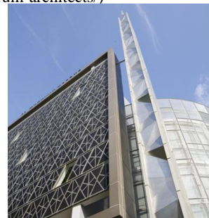
Fig. (3.85): Detail view of the façade screens. (Source: http://islamicprojects.wordpress.com/2011/07/29/al-mukminin-mosque-forum-architects/ )
